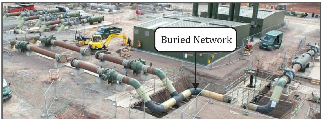
Figure 2.29: Construction and installation of an underground pipe network being lay down before burial. [24].
