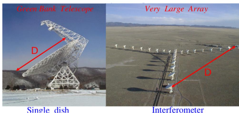
Figure 2.4: Diameter for a single dish and distance for an interferometric system (baseline).
