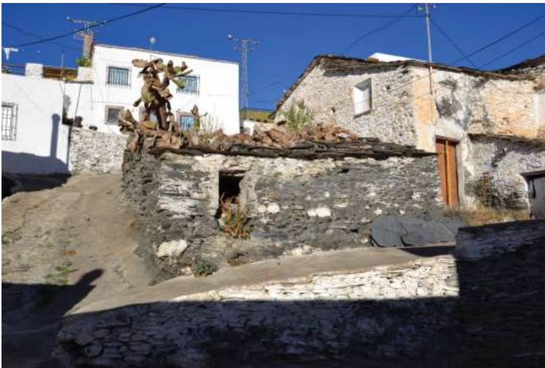
Fig. 2.1. A dead chumbera (prickly pear) emerges from a collapsed roof.
