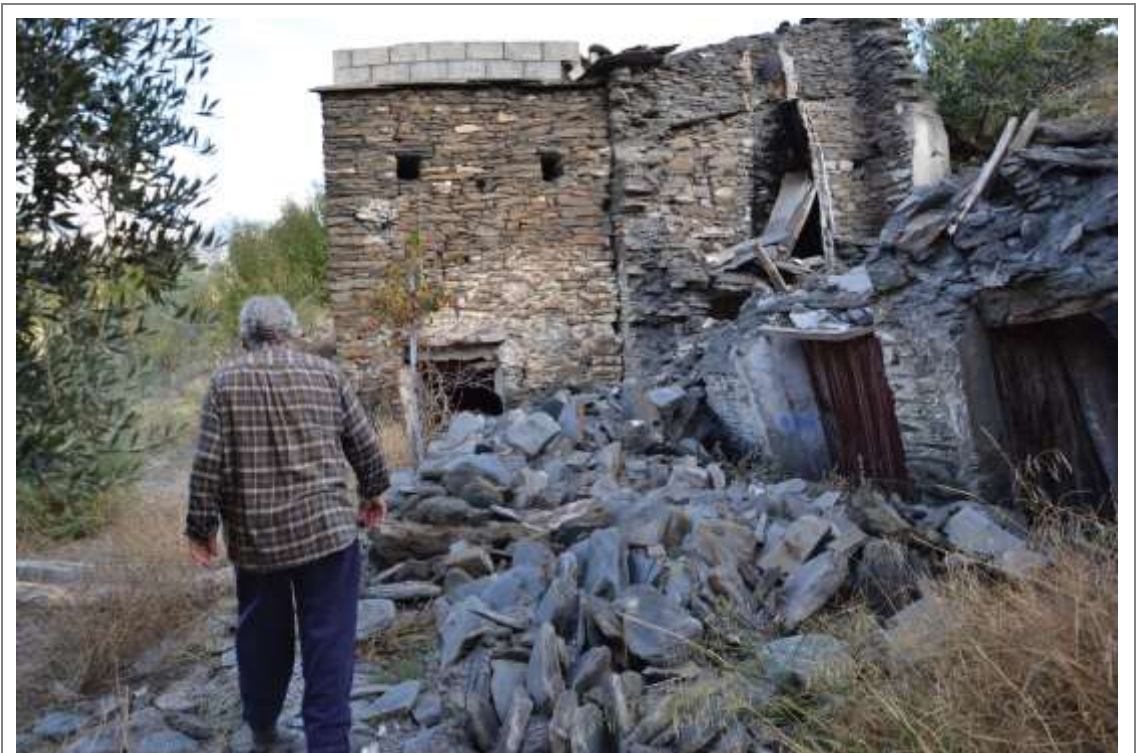
Fig. 2.4. Villager walking by a collapsed cortijo .
