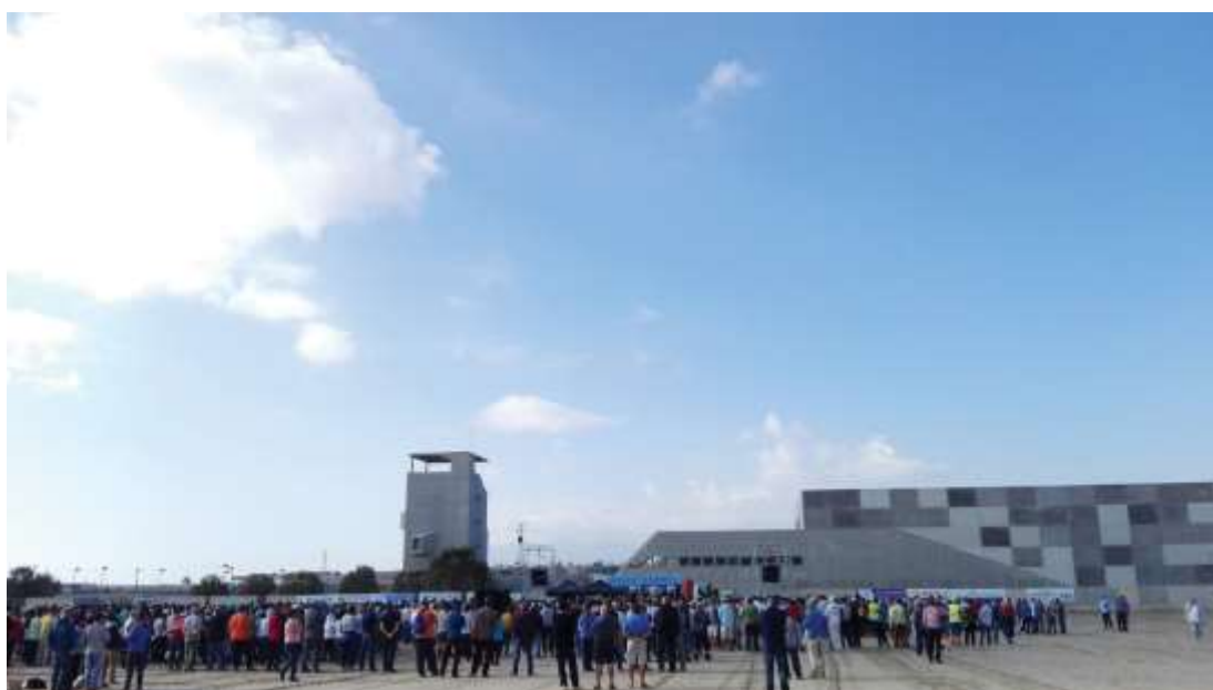
Fig. 3.9. Some 4,000 farmers gathered in front of the futurist Bajo Almanzora desalination plant on 16 October 2017 to demand its immediate repair.
