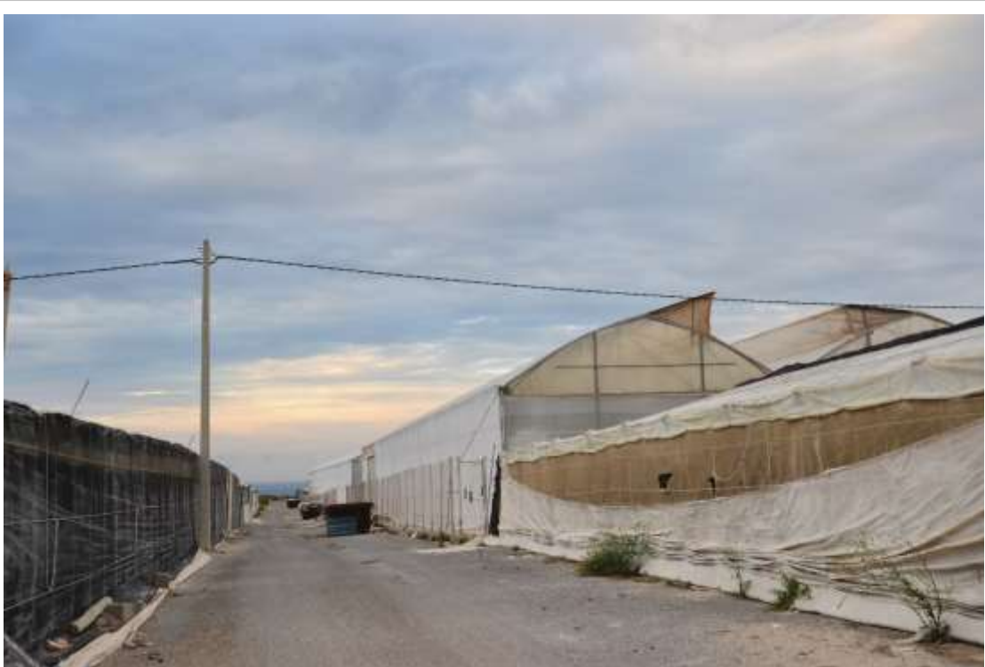
Fig. 3.6. Different greenhouse models built next to each other: ‘raspa y amagado’ in the front and to the left; the taller ‘multitúnel’ in the back.
