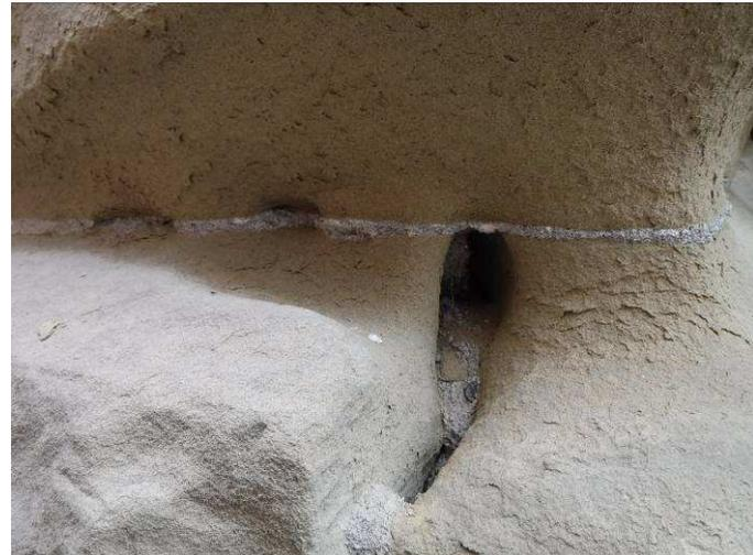
**Plate No. 3:** Close-up of eroded stone and bedding mortar
