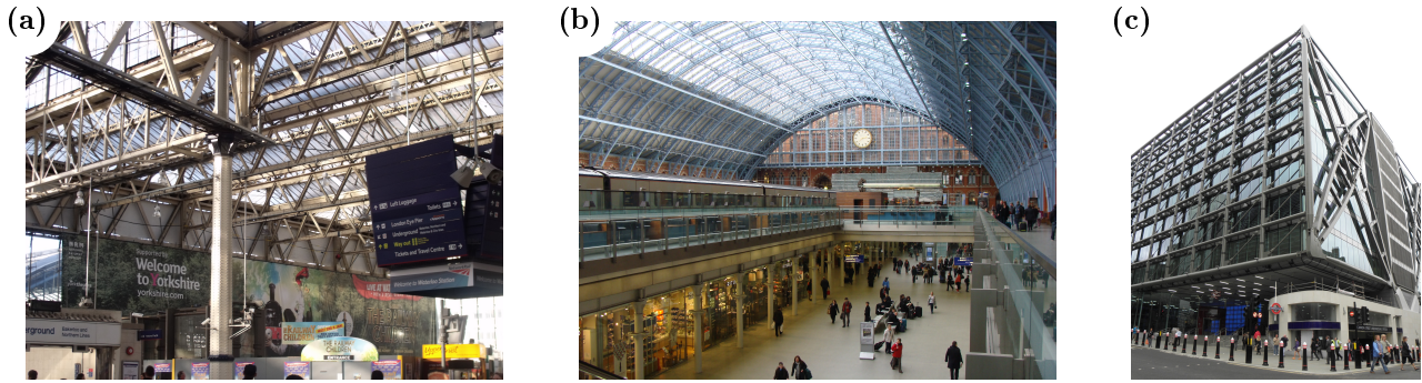
Figure 1.2: Three railway stations in London, each with different structural forms. (a) Waterloo station, showing a series of Warren trusses of varying depth (photo by Brown, 2011, used under CC BY 2.0). (b) St Pancras International station, with arched roof vault (photo by Sakrajda, 2010, used under CC BY-SA 3.0). (c) Cannon Street station with Cannon Place office block above, the exoskeleton of the office block comprises transfer trusses, using Pratt trusses and cross braced cantilever layouts (photo by Prasannan, 2012, CC BY-SA 3.0).
