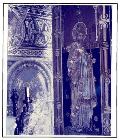
Paraged wallpaintings in the nave of the church at Garton-on-the-Wolds, East Yorkshire. The losses are most serious on the inside of the exterior wall and the contiguous interior cross wall due to penetration of moisture.
