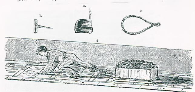
The candle-holder: a socket of iron, having a spike at right angles for the convenience of sticking the light in the sides of the pit when stationary. The spike also forms a handle when the light is carried before them.
