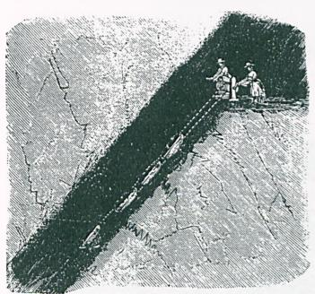
Sectional View of Diagram No. 1, with Girls winding Coal from the Workings in the Dip.
