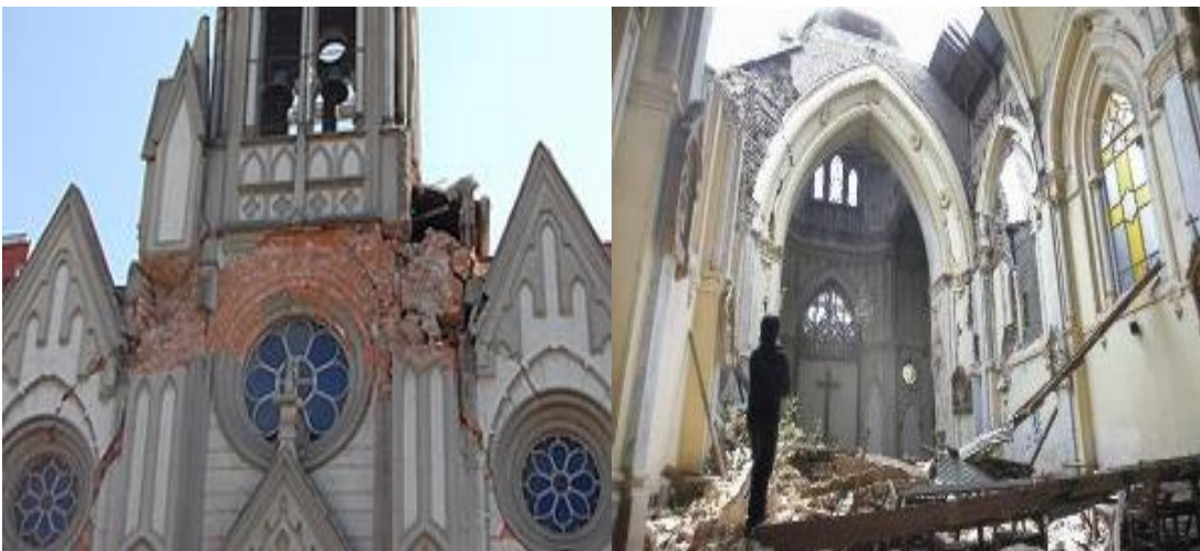
Image 54: The state of disrepair post-2010 Earthquake of the Twelve Apostles Church. This was one of the first churches ever built in the city. Source: PlataformaUrbana.cl (2015).
