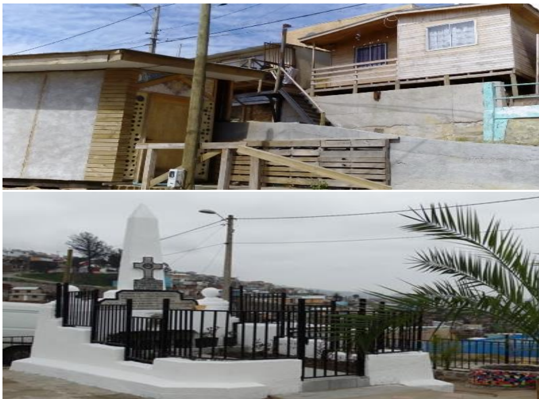
Image 19: House built on another house.
