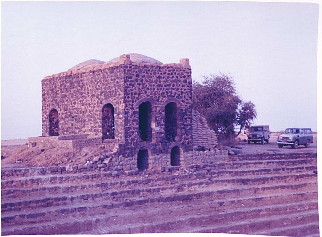
2. Guard-house built between the settling tank and main cistern with two sluice-ways underneath,
