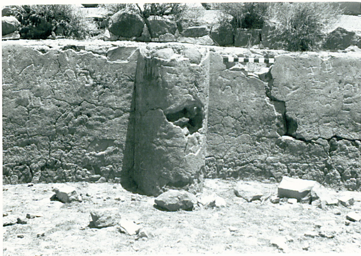
2. Close-up of the interior of Birkat Uraynibah showing thick covering of plaster.
