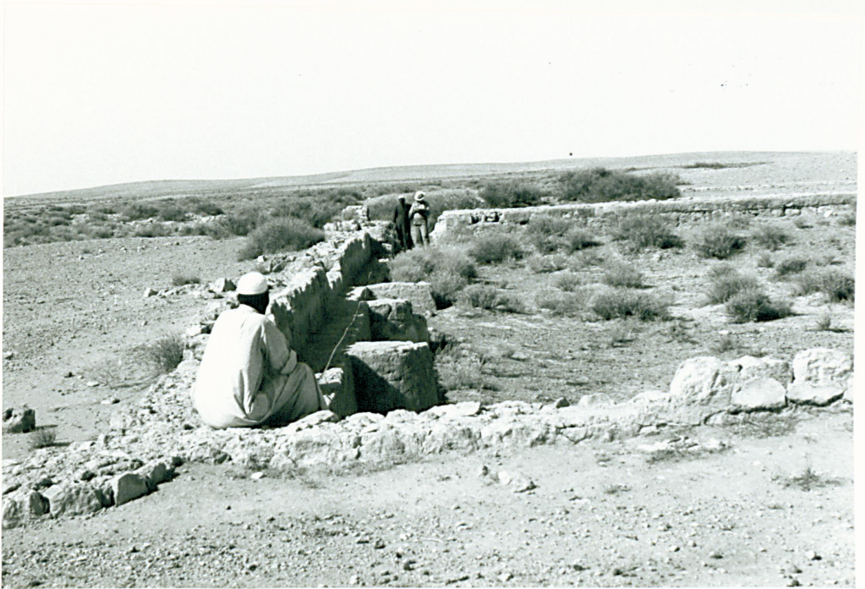
1. Birkat ath-Tha'labīyyah showing main tank and inlet in background,
