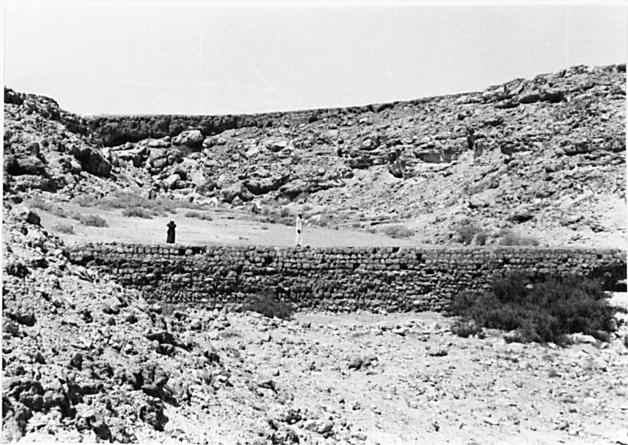
2. Close-up of the dam as seen from the south. It has suffered slight damage.
