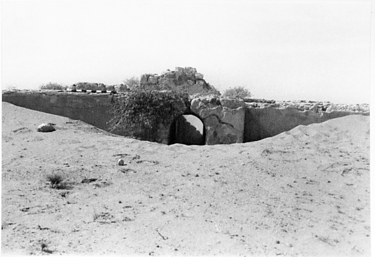
2. Close-up of the inlet with original plastering on interior of birkah.
