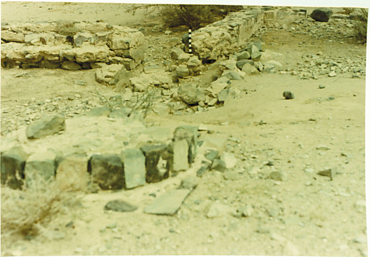
1. Close-up of buttress on the exterior of the western wall of Birkat al-Mislah.
