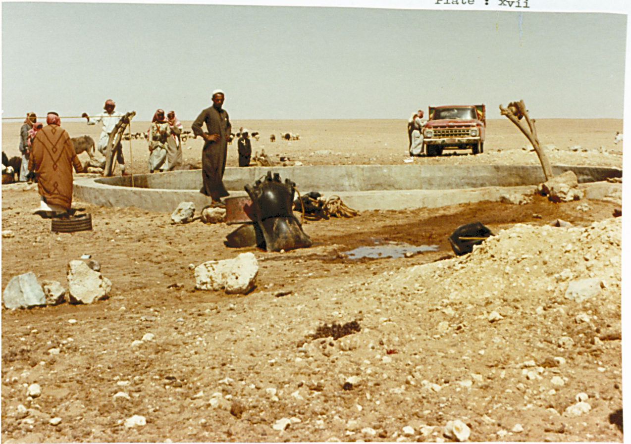
1. Well of al-Bid'. It has been repaired and contains fresh water.
