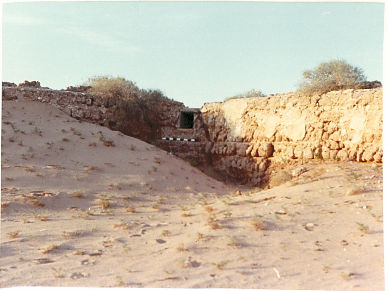
2. View of mouth of channel at the north east corner, original plastering visible.
