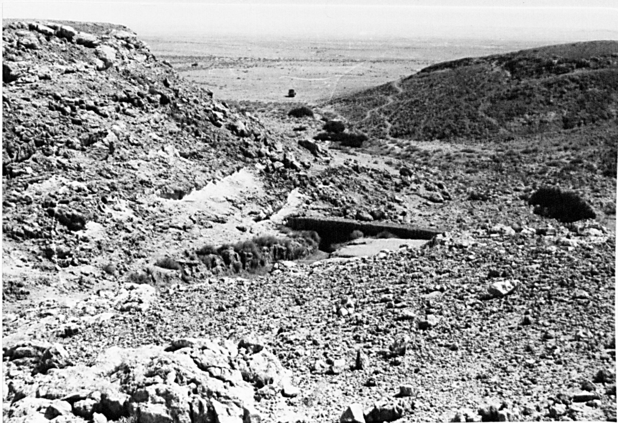
1. Dam of al-'Aqabah across ravine at Sha'Ib al-Batn.
