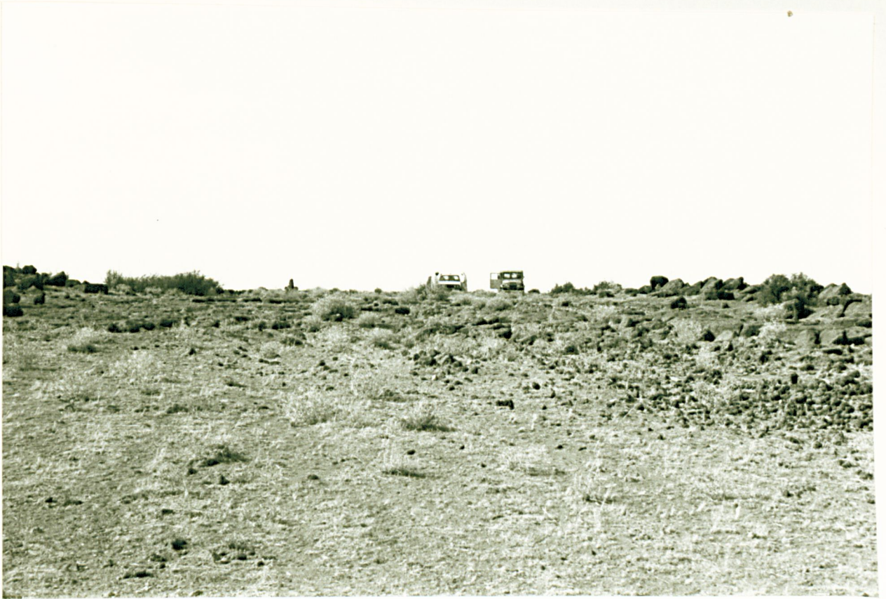
1. 2 km. south of Fayd the road had to be cleared and widened for ca. 18 metres.
