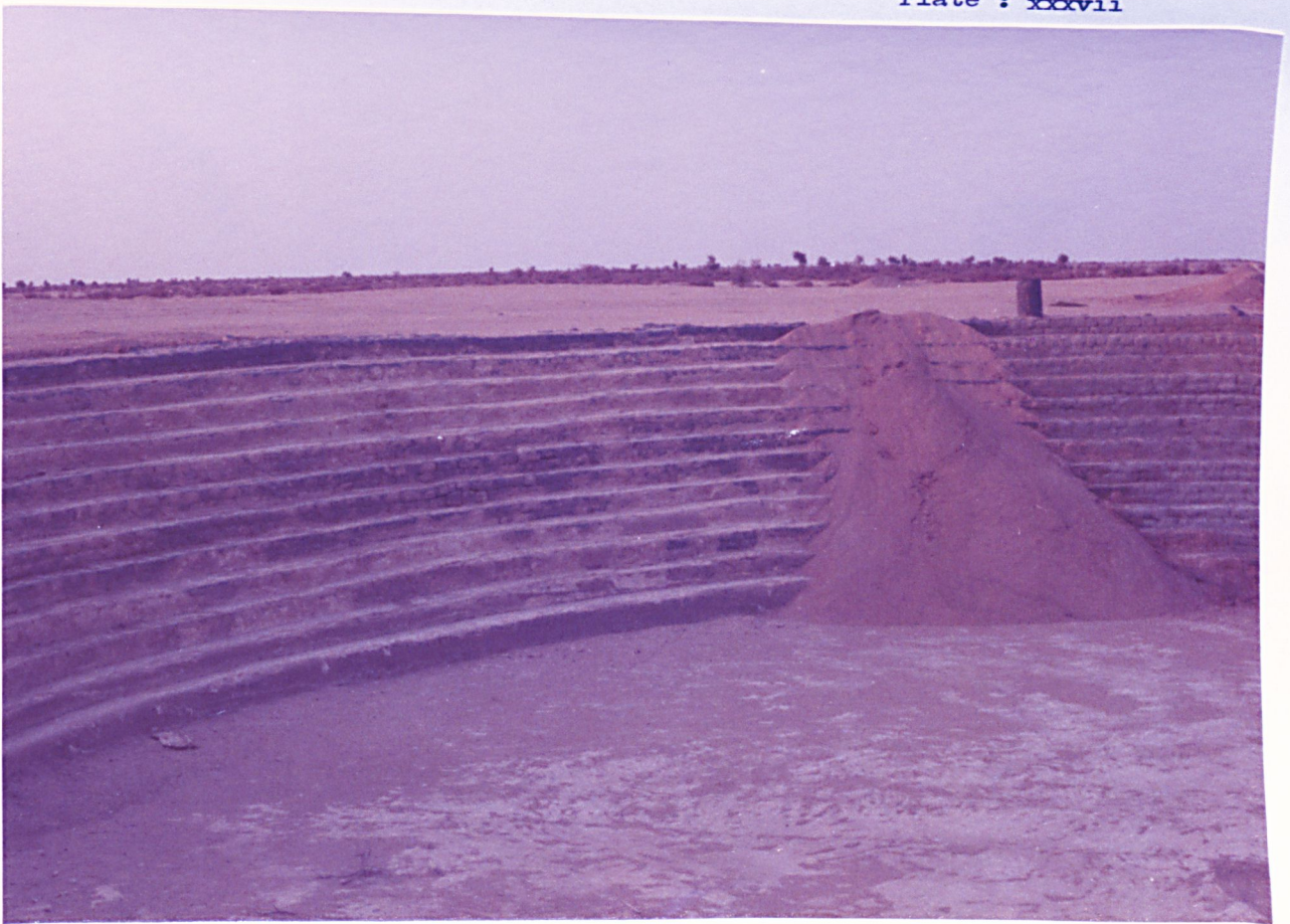
1. Birkat al-Kharābah: the main tank after clearing it showed a depth of 5.84 m. and diameter of ca. 54 m.
