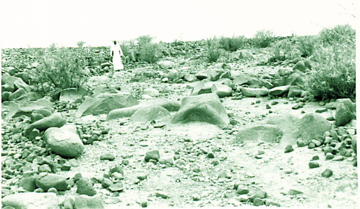
2. The road in very rough areas was sometimes divided into two lanes by immovable boulders.
