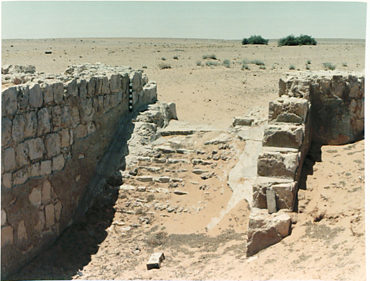
2. Details of inlet, with sloping channel, which was formerly covered with a layer of lime.
