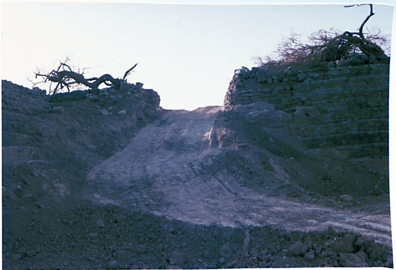
1. In cleaning the birkah a bulldozer was used, causing considerable damage.
