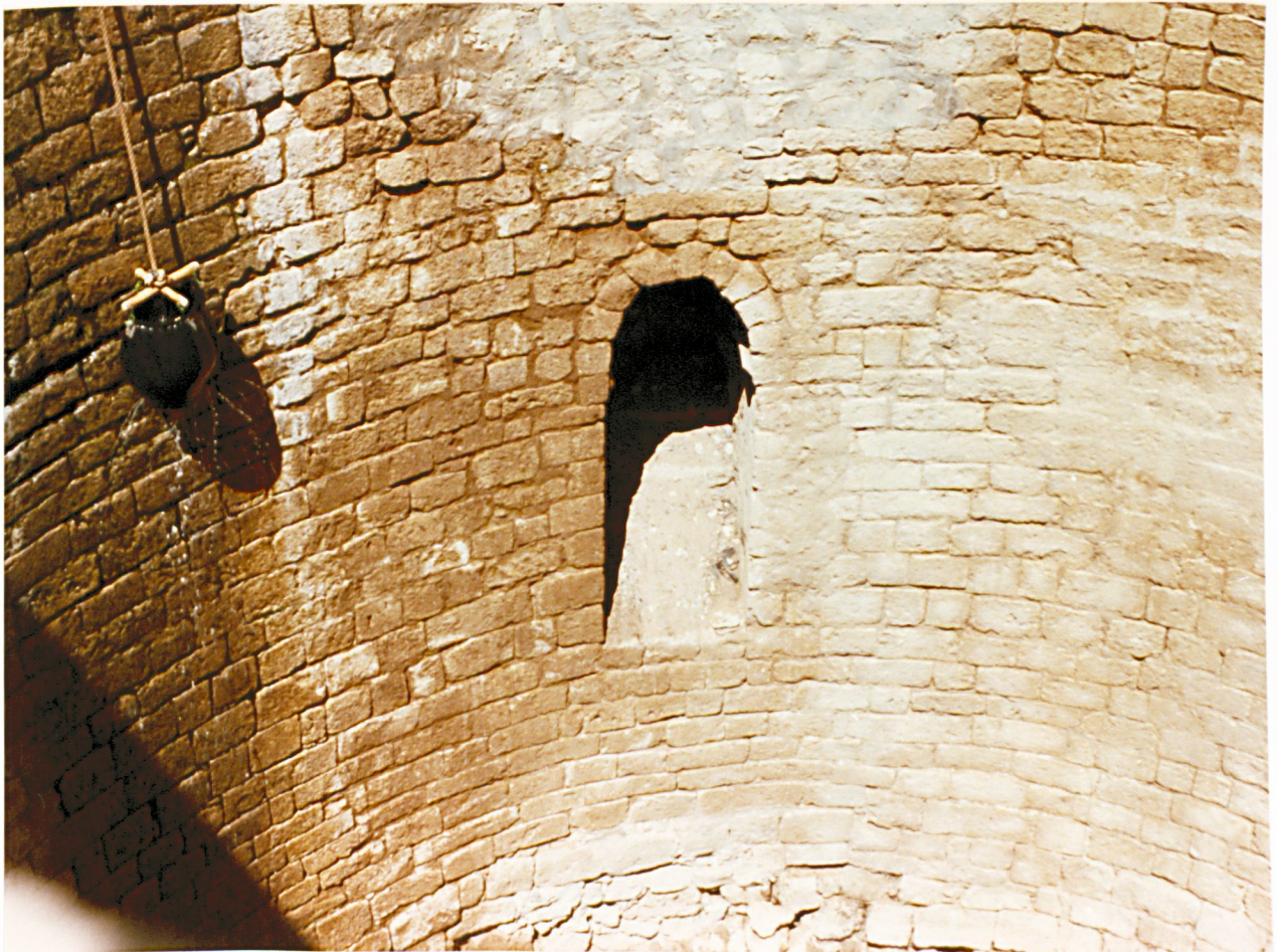
2. Lower section of well showing neat lining of roughly cut stone, with small opening just above water level.
