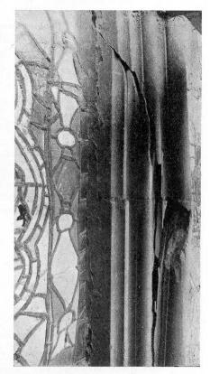
Example of Exterior decay in parts, Tracery and Mullions of Chapter-House fractured by expansion of the iron saddlebars, now restored.
