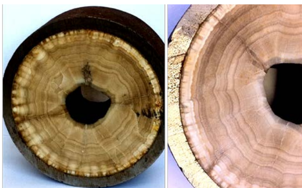
Figure 3.3: Calcium carbonate deposits in oil and gas pipes – Sample provided by private communication with BP, Sunbury, UK.
