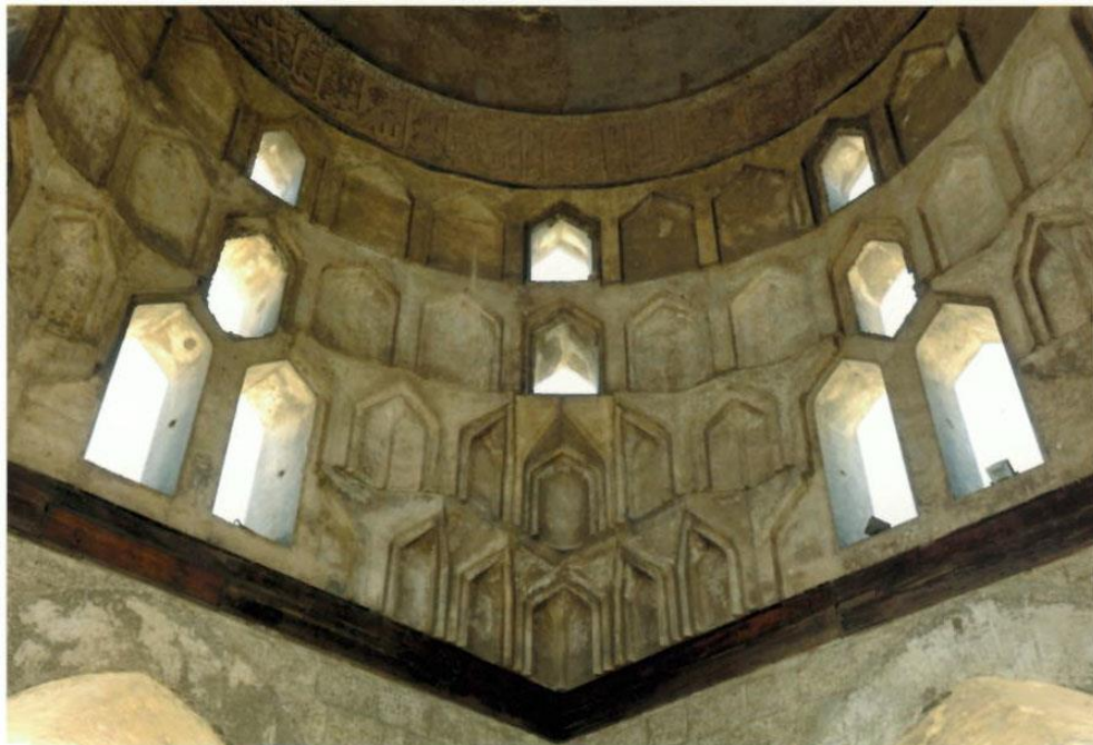
Figure 80, Interior of the Fisqiya showing the system of squinches that supports the dome, Mosque of Ibn Tulun, Cairo. From: Swelim, Ibn Tulun , 78.
