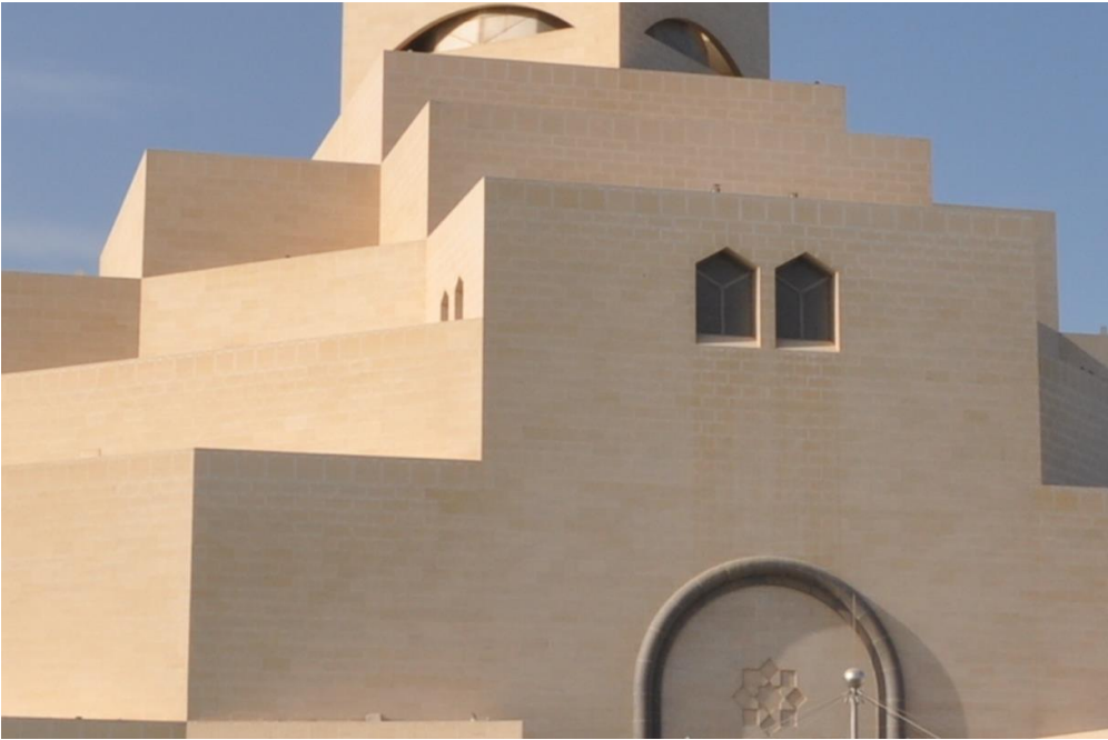
Figure 77, Detail of architectural façade of the MIA.
