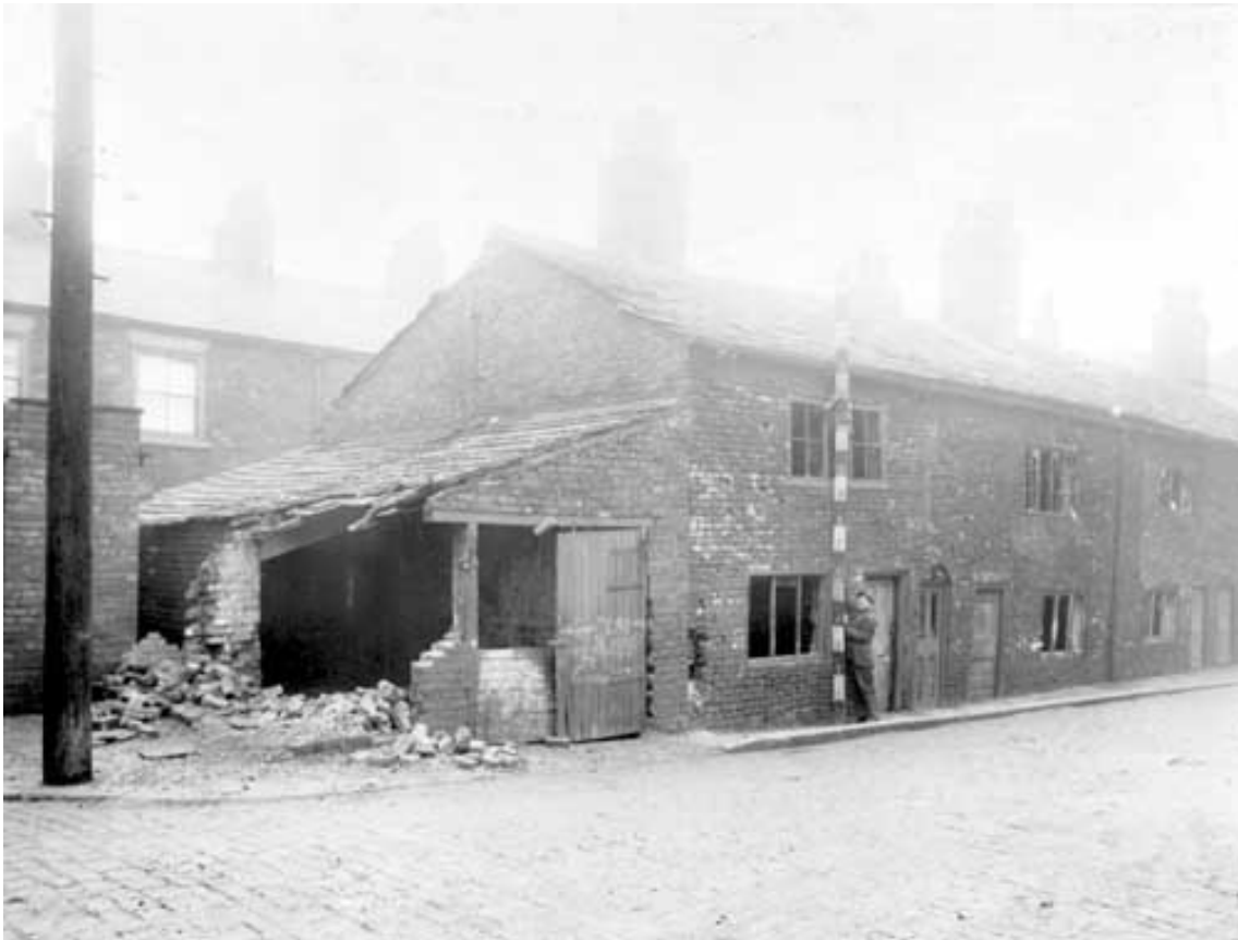
Figure 6.9 Housing in Czar Street, Holbeck, photographed just prior to demolition in 1915
