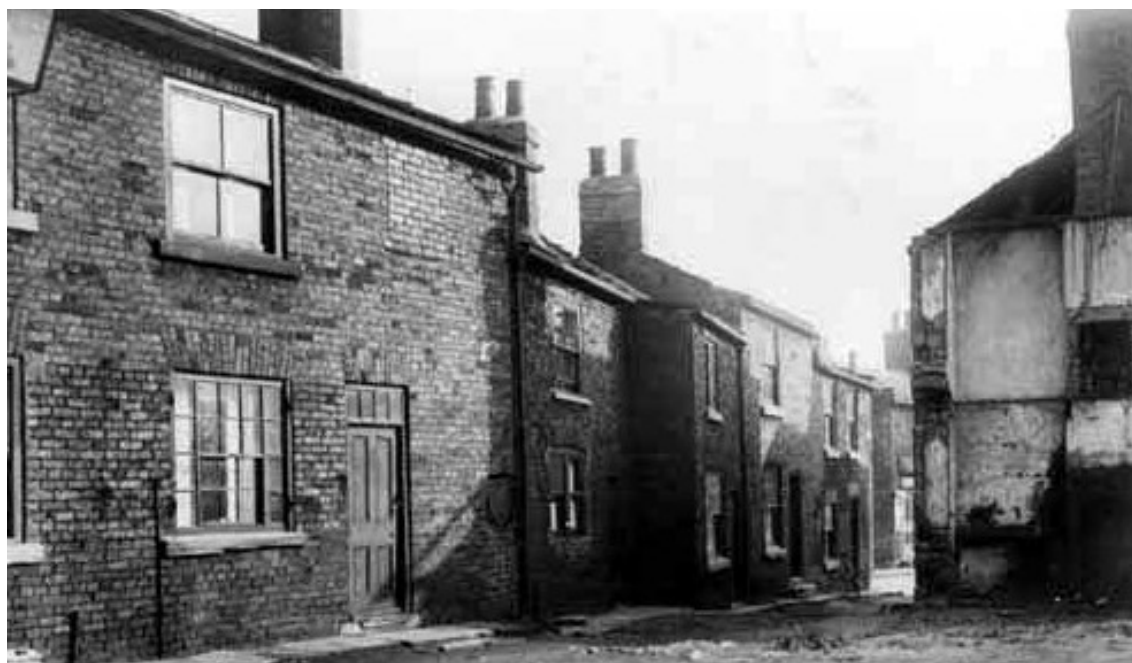
Figure 3.6 Two photographs of Woggon Yard, Rothwell, prior to demolition in 1935
