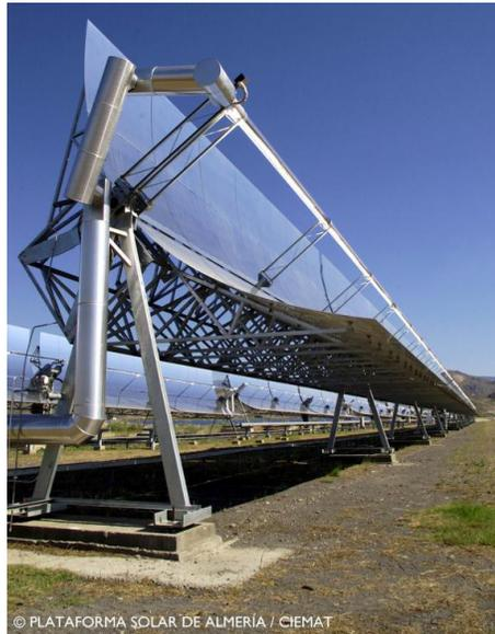
Figure 2.1: ACUREX distributed solar collector field.
