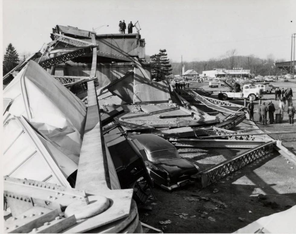
**Figure 1-1** Silver Bridge after collapse showing the Ohio side of river<sup>5</sup>
