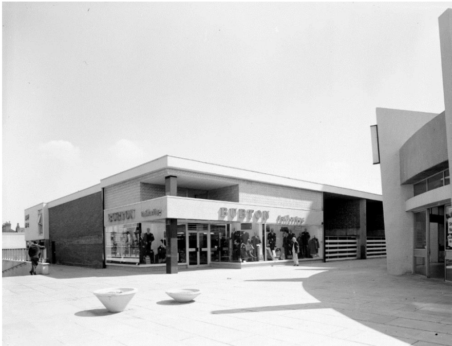
2.19 Exterior of a new Burtons branch in an unidentified shopping precinct, 1968. LMG, LEEDM.P.2003.1.0190.
