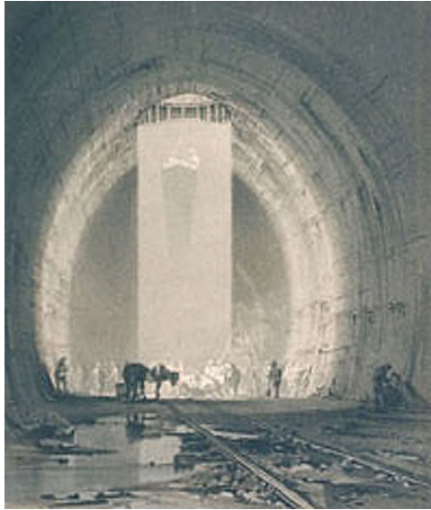
26. Kilsby Tunnel: working shaft J. C. Bourne London Science Museum
