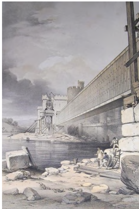
4. Menai Straits Tubular Bridge, Edwin Clark, 1850 Engraving shows one tube in place.
