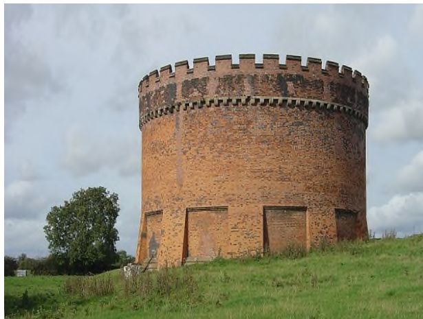
63. Kilsby Tunnel, brick ventilation shaft. Private photo
