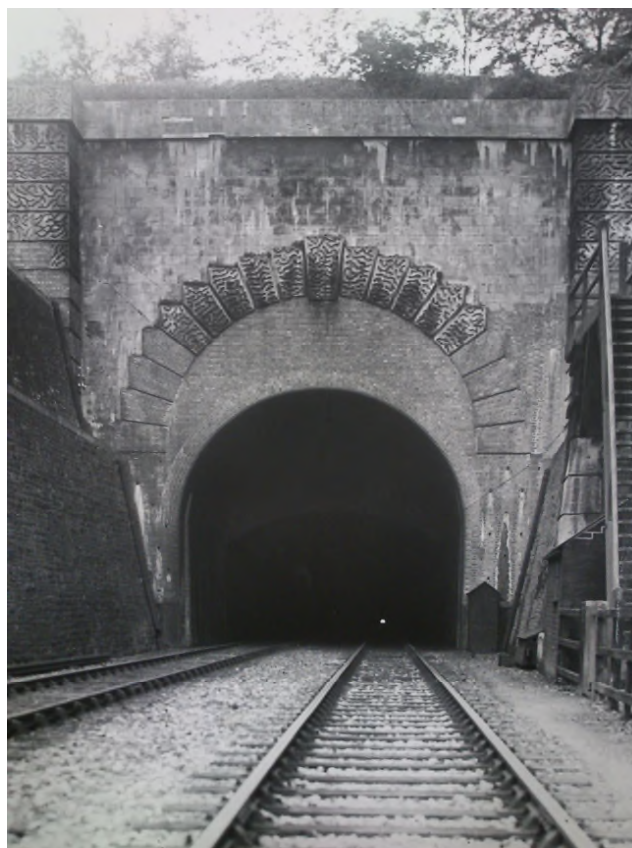
91. This photograph of the eastern portal shows clearly the original dimensions of the arch which has been decreased by the inseting of a smaller arch in brick. The entrance to the stone quarry is on the right. Leicester University, Edgar Randall Collection, vol. 6 B5609
