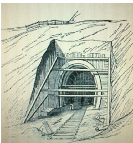
3. Method of timbering the face of the excavation at the intended entrance of Saltwood Tunnel, Kent.
