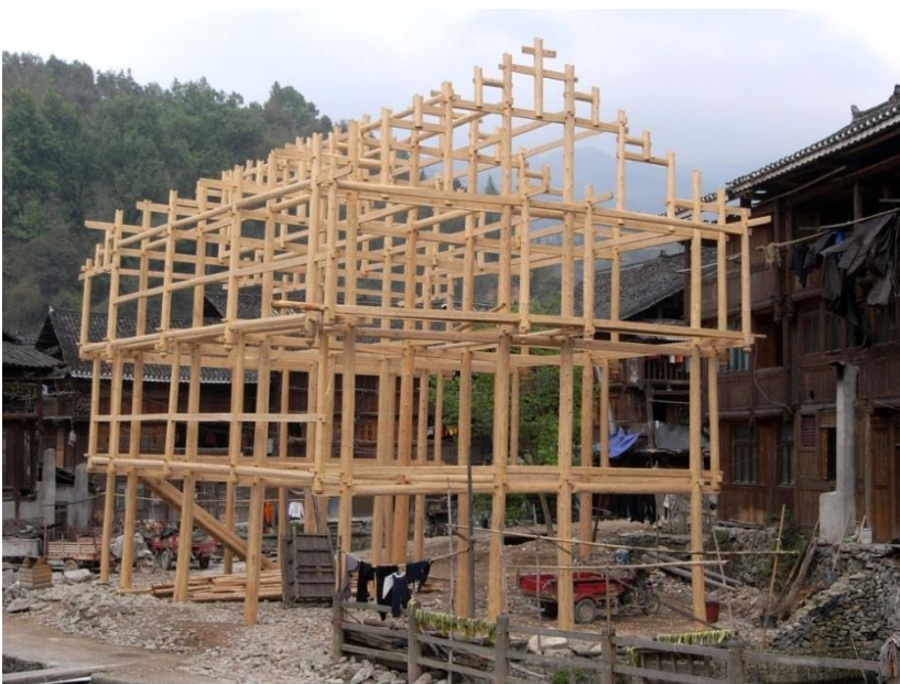
Figure 9. Column-and-tie structure, at Zhaoxing village. Photograph by Derong Kong.
