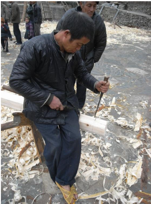
Figure 89. Carpenter uses an axe as hammer. Photograph by Derong Kong.
