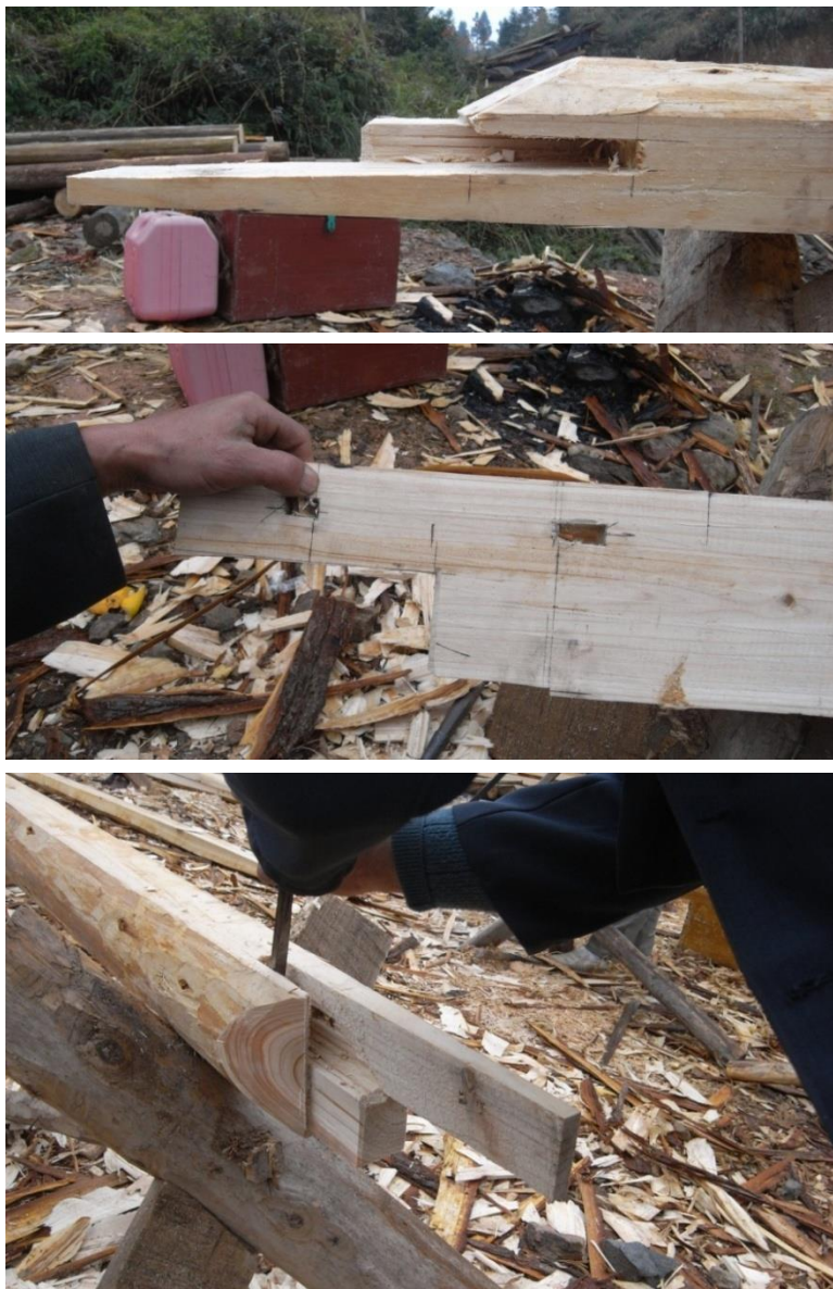
Figure 56. An interlocking tenon made by the carpenter Wendong Lu, at Xiaohuang village, 2010. Photograph by Derong Kong.
