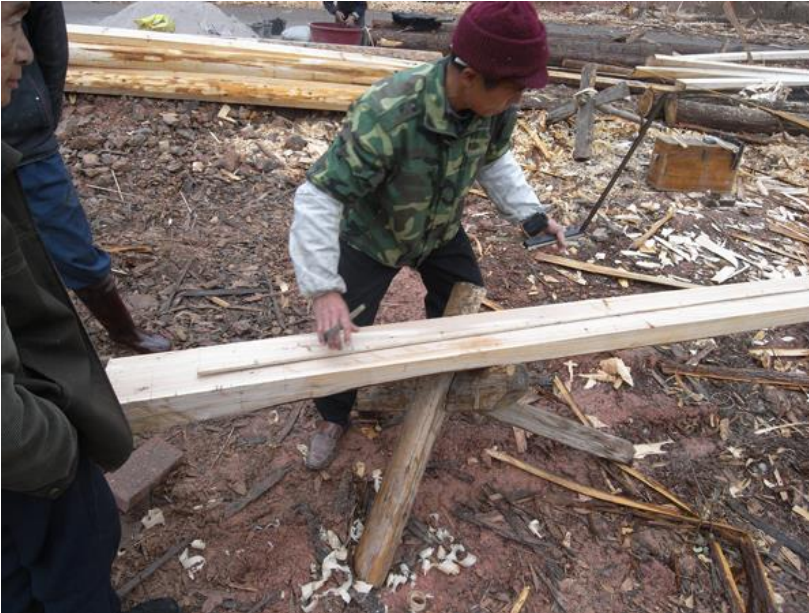
Figure 12. The hand-ink master Yongcheng Lu draws an ink line on a component. Photograph by Derong Kong.
