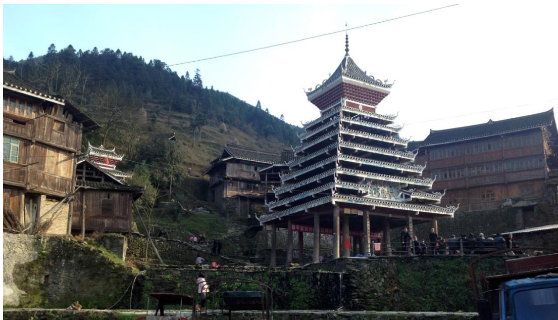
Figure 36. Dense eaves style, Tang'an. Photograph by Derong Kong.
