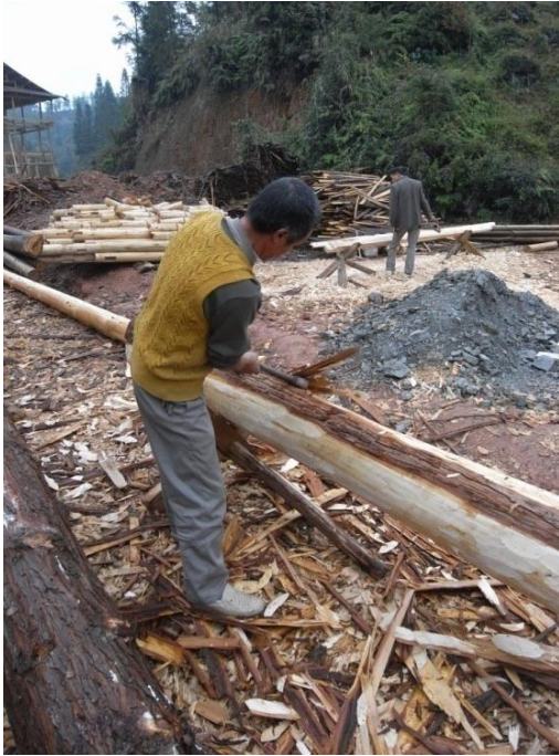
Figure 8. Removing the tree bark.
