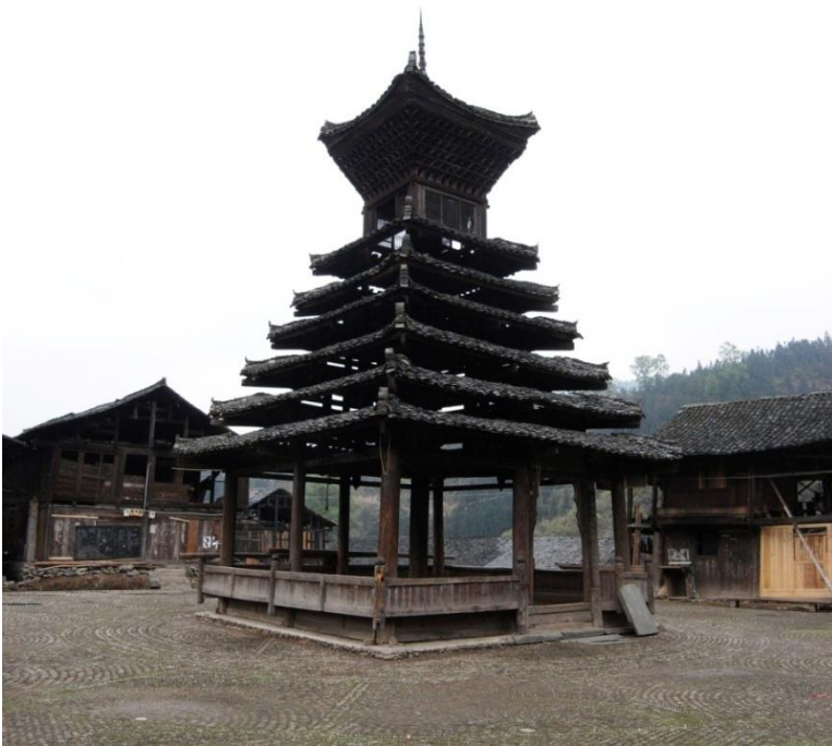
Figure 40. Single column tower at Shudong village in Liping County. Photograph by Derong Kong.
