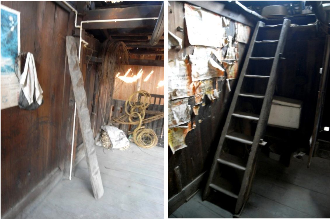
Figure 25. The ladder and stair to loft. Photograph by Derong Kong.
