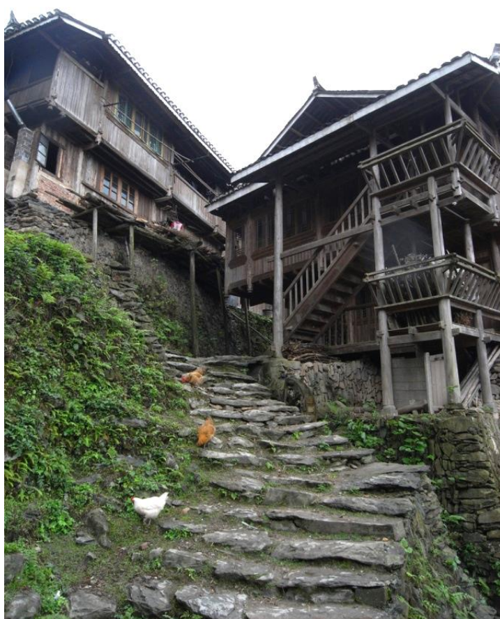
Figure 7. Ganlan building, at Tang'an village. Photograph by Derong Kong.
