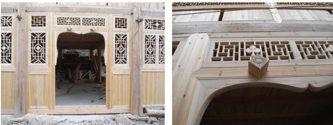
Figure 26. Door and door hammer. Photograph by Derong Kong.
