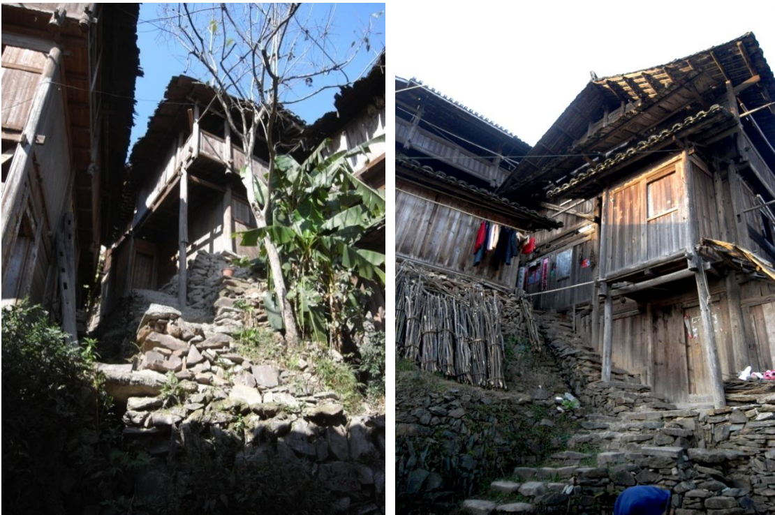
Figure 5. Ganlan building, Dong house. Photograph by Derong Kong.
