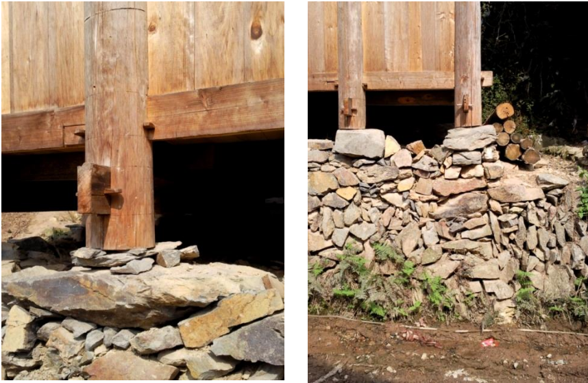
Figure 10. Column base. Photograph by Derong Kong.
