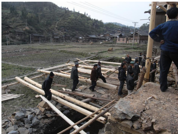
Figure 20. Pre-assembling components at Xiao Huang village, 2010, in Congjiang County, Guizhou Province. Photograph by Derong Kong.
