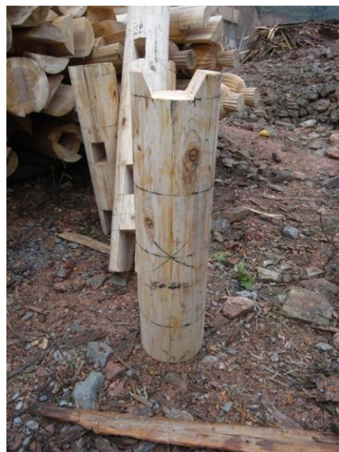
Figure 12. The hand-ink master Wenli Lu's carpenter code on the fifth row of the front second short column. Photograph by Derong Kong.
