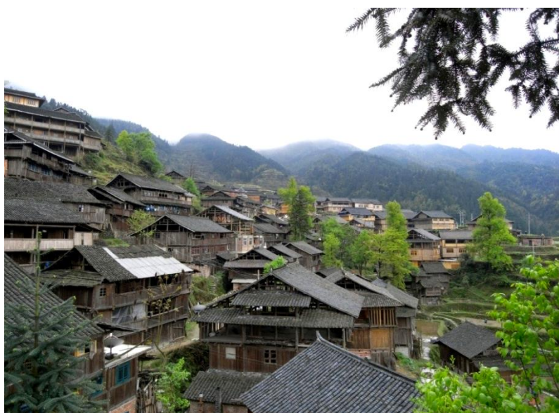
Figure 5. Ganlan Building, at Tang'an village. Photograph by Derong Kong.
