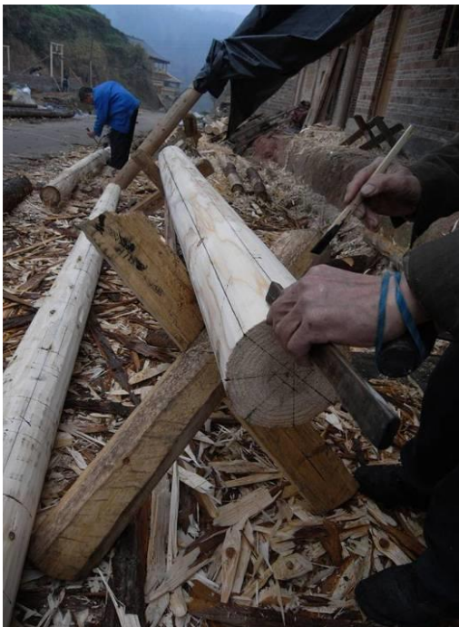
Figure 8. Removing the tree bark.
