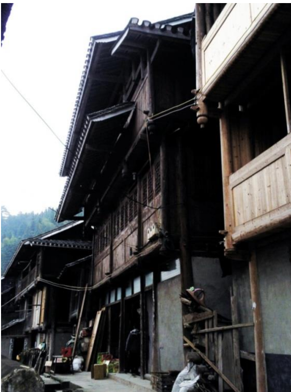
Figure 34. The double eaves. Photograph by Derong Kong.
