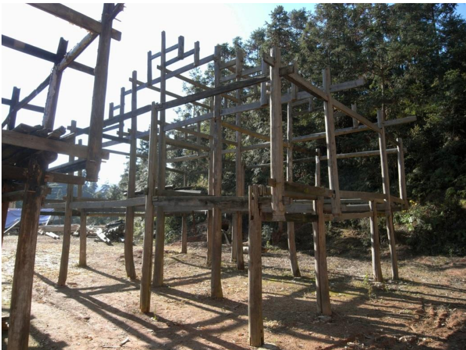
Figure 23. An abandoned house structure. Photograph by Derong Kong.
