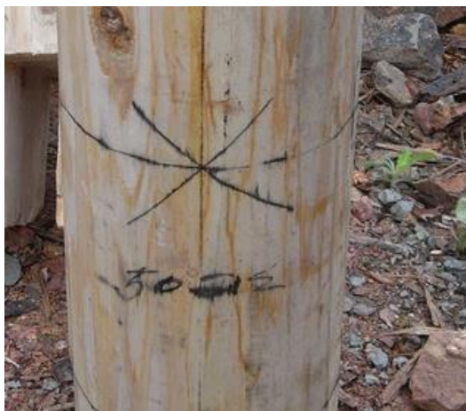
Figure 12. The hand-ink master Wenli Lu's carpenter code on the fifth row of the front second short column. Photograph by Derong Kong.
