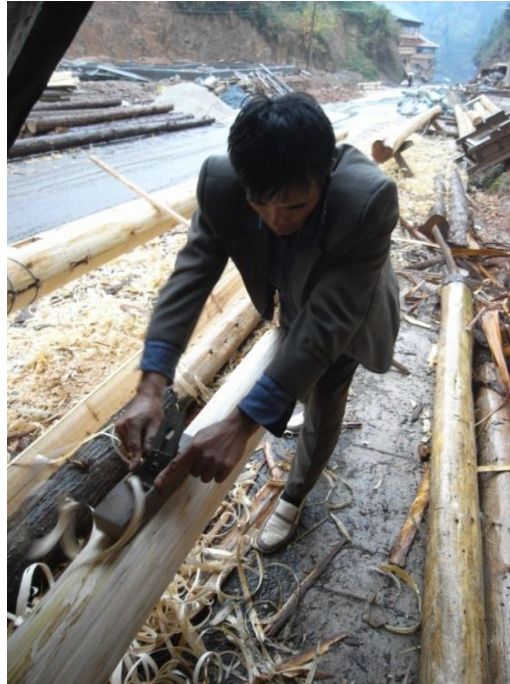
Figure 9. Planing the surface of the timber.
