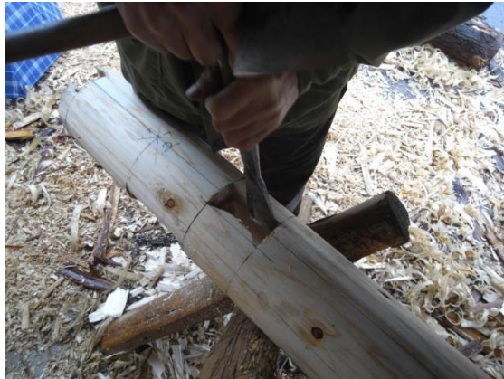
Figure 11. Chiseling the mortises on the column. Photograph by Derong Kong.
