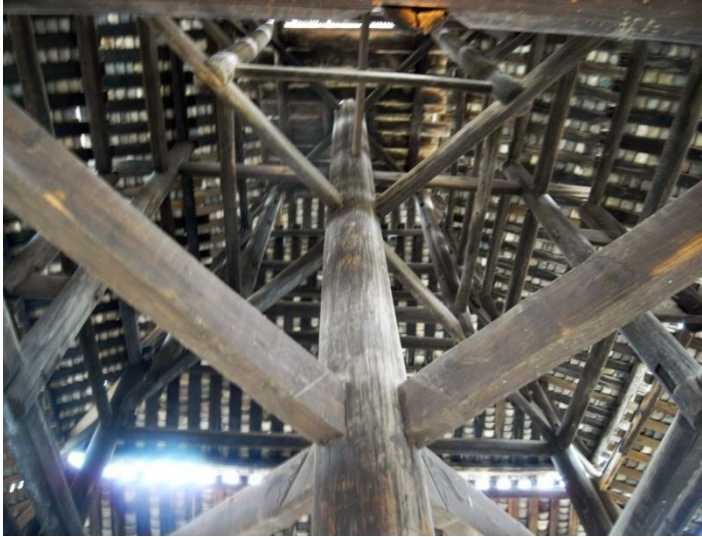
Figure 41. The central column of Shudong single column tower. Photograph by Derong Kong.
