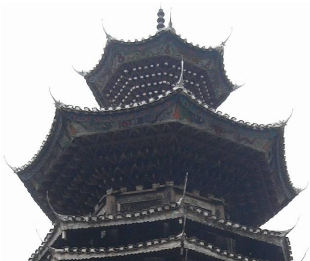
Figure 15. The desirable-bracket-set, at Zengchong village. Photograph by Derong Kong.
