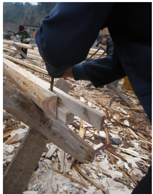
Figure 14. The hand-ink master Wenli Lu draws ink lines on draft wooden components. Photograph by Derong Kong.
