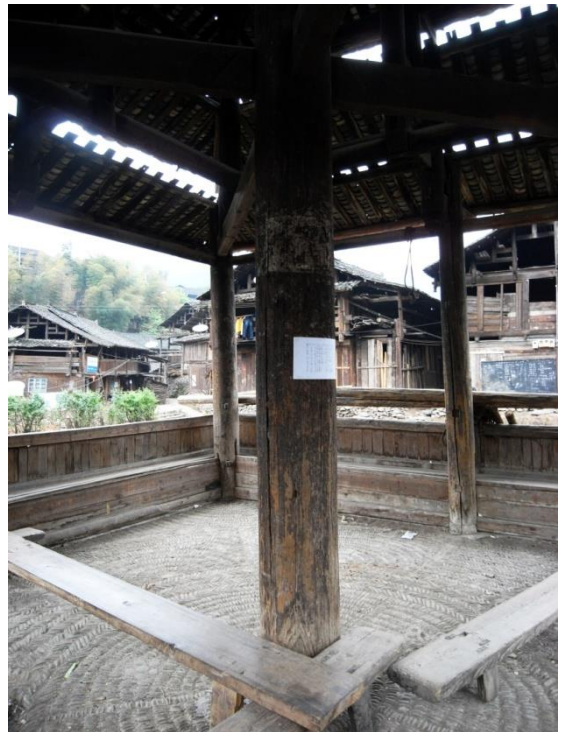
Figure 42. The structure of Shudong single column tower. Photograph by Derong Kong.
