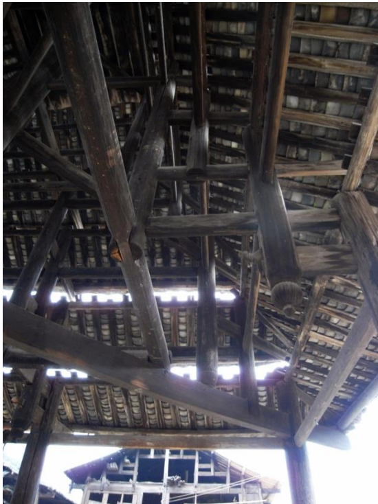
Figure 42. The structure of Shudong single column tower. Photograph by Derong Kong.
