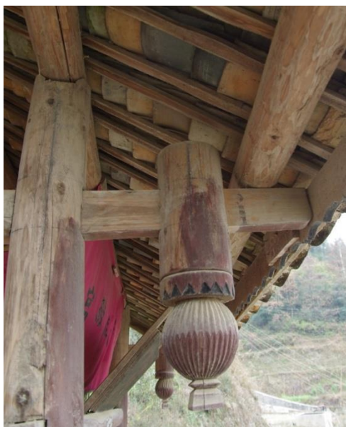
Figure 61. The hard-tenon in the structure of an earth altar, at Guima village, 2014. Photograph by Derong Kong.
