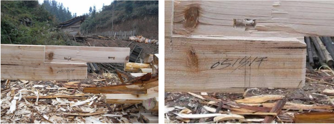
Figure 18. The hand-ink master Wenli Lu's carpenter code on the back fifth row of the first tie-beam to connect with the first hanging column. Photograph by Derong Kong.
