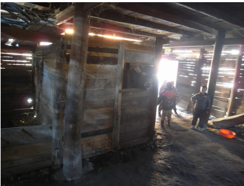
Figure 5. Ground floor. Photograph by Derong Kong.
