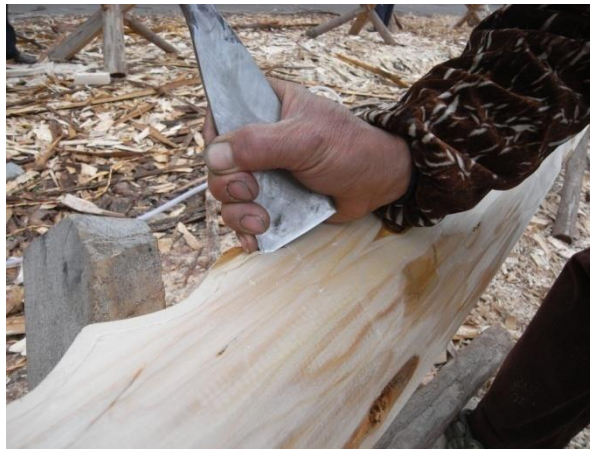
Figure 88. Carpenter uses a chisel to carve timber. Photograph by Derong Kong.
