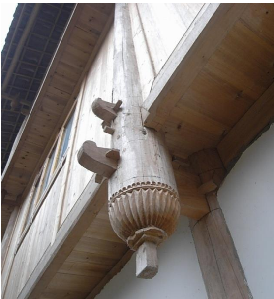
Figure 58. The half-tenon in the hand-ink master Wenli Lu's house, at Luoxiang Town, 2013. Photograph by Derong Kong.
