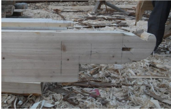
Figure 59. A finished half-tenon, at Xiaohuang village, 2010. Photograph by Derong Kong.
