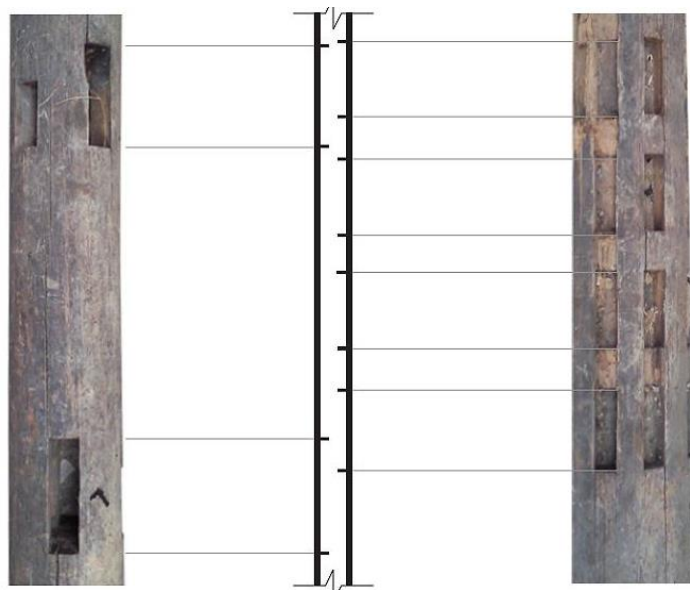
Figure 74. Diagram of sizes on a Zhang pole transferred during construction. Photograph and drawing by Derong Kong.
