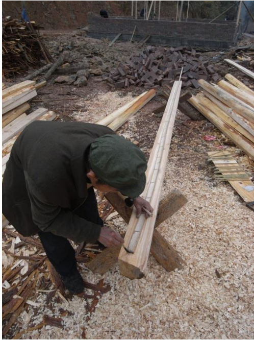
Figure 14. The hand-ink master Wenli Lu draws ink lines on draft wooden components. Photograph by Derong Kong.
