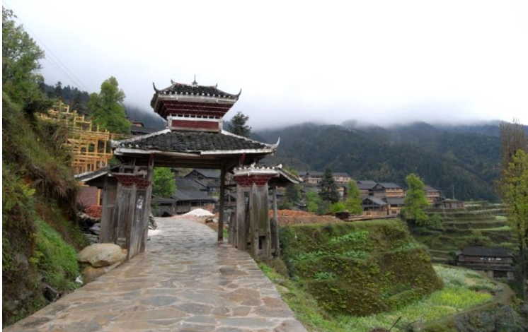
Figure 30. The main gate of Tang'an village. Photograph by Derong Kong.
