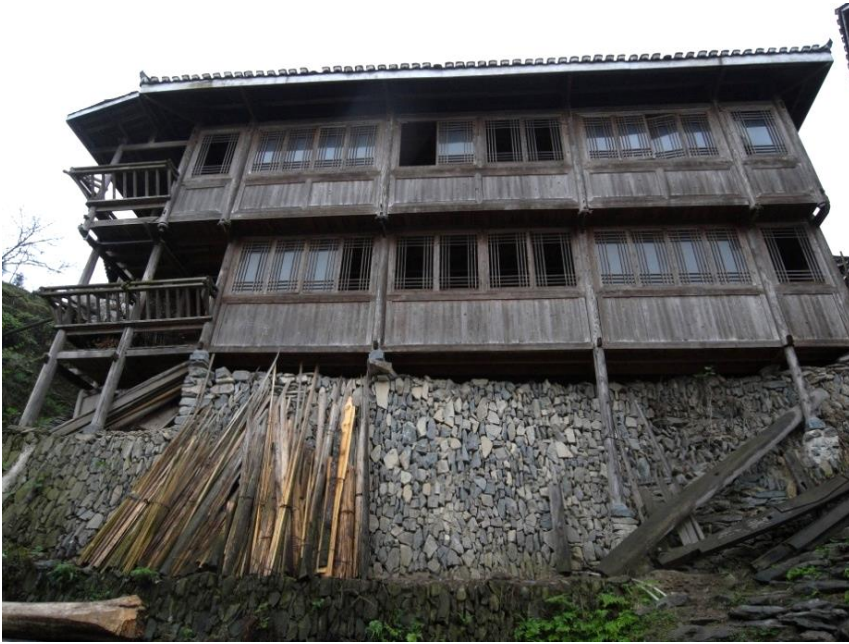
Figure 8. Ganlan building, at Tang'an village. Photograph by Derong Kong.
