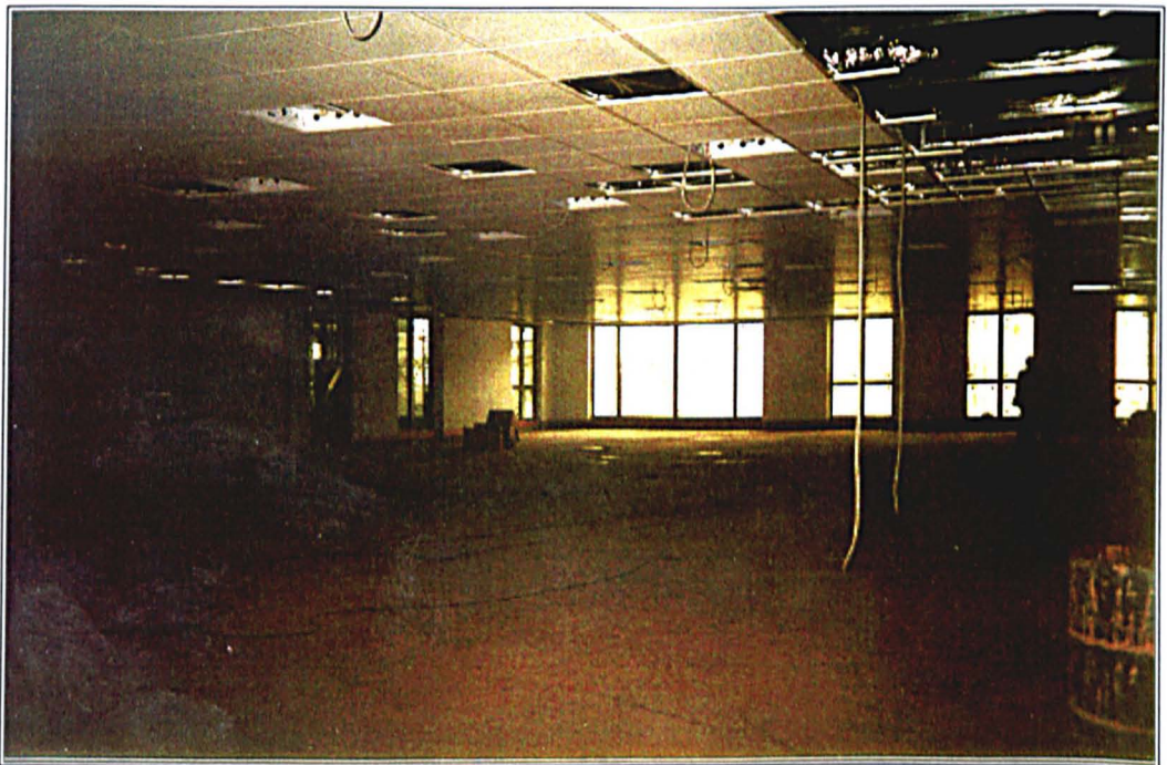
Figure 4.2: Test Structure A (Configuration 1) - Photograph.
