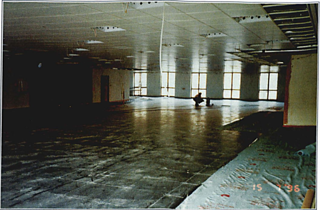
Figure 4.47: Structure A (Configuration 2) - General View.
