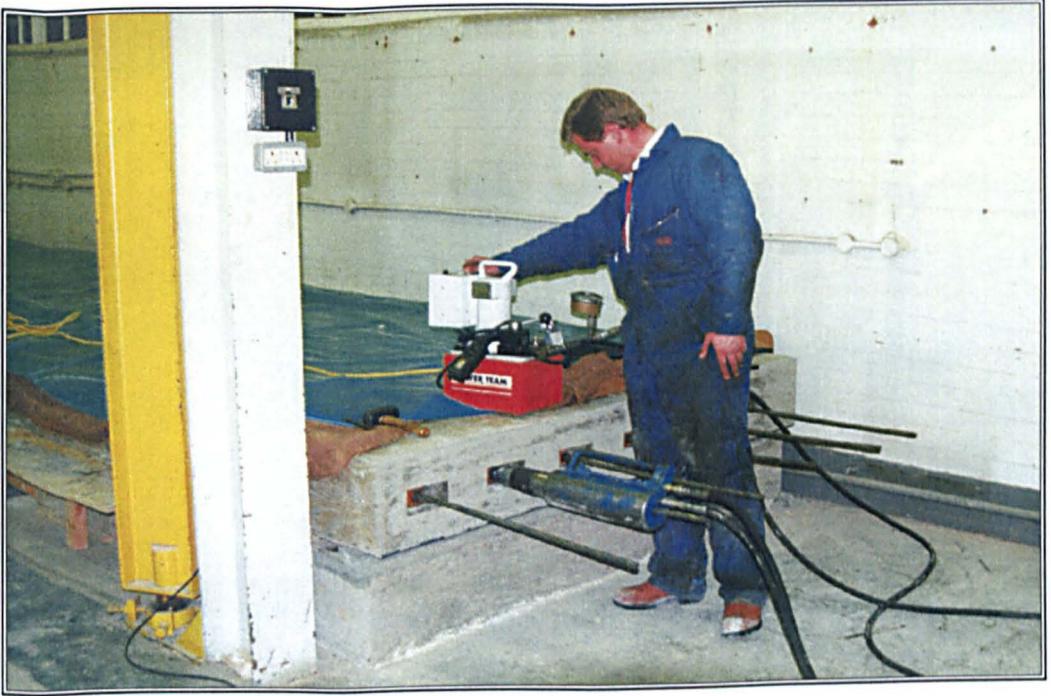
Figure 4.74: Structure C - Post-Tensioning in Progress.
