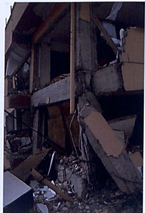
**Figure 1.3 Partial building collapse due to severe damage in beam-column connections after the 1999 Izmit, Turkey earthquake, (NISEE, 2012)**
