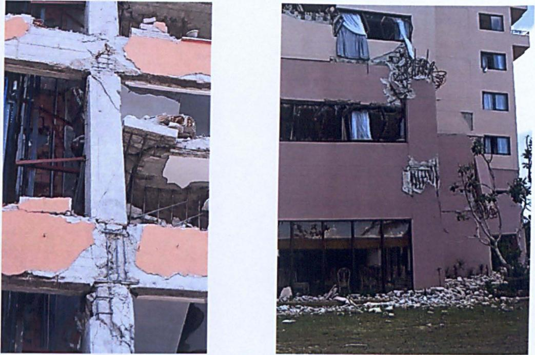
**Figure 1.4 Observed damage in deficient beam-column joints (Moehle, 2008)**
