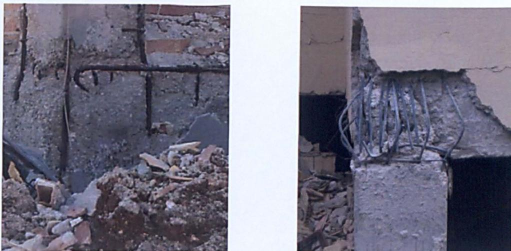
**Figure 1.5** Deficient beam-column joints, 2009 L'aquila, Italy earthquake (Verderame et al., 2009)
