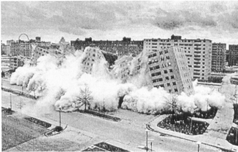
[Fig. 33] Demolition of Pruitt-Igoe apartment blocks in 1972
