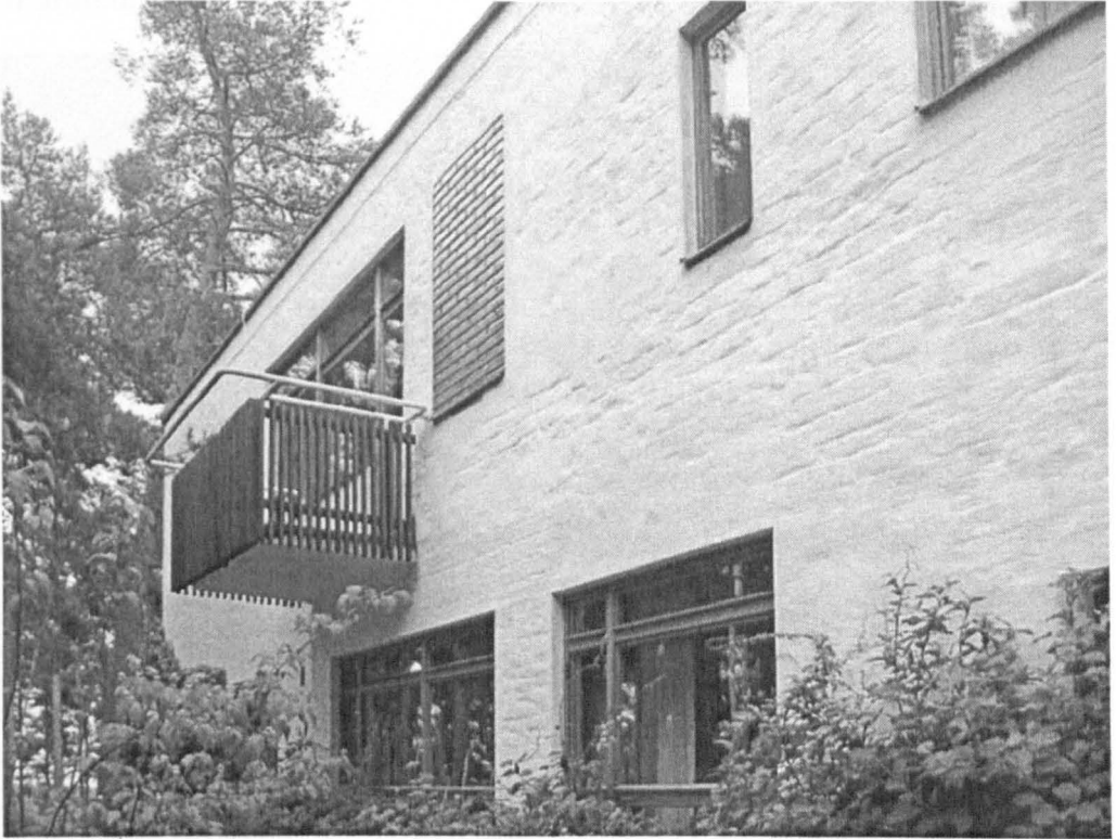
[Fig. 5-78] Different reliefs on whitewashed walls: uneven finish of northeast façade (top) and interior wall of living room that clearly reveals the brick layers (bottom)
