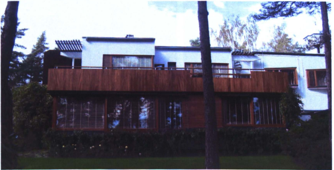
[Fig. 5-76] White plastered exterior wall partly guarded by timber cladding masses
