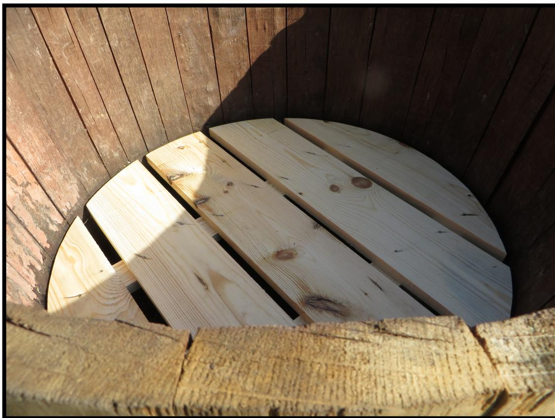
Figure 5: wooden boards to prevent tap blockage
