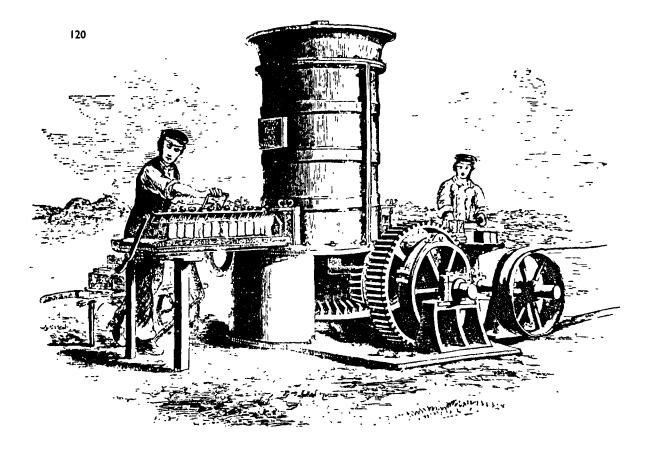
Figure 7.1. Extrusion brickmaking machine attached to a pug mill, Bulmer and Sharp, manufacturer, c.1860. [From John Woodforde, <u>Bricks to Build a House</u> (1976)]
