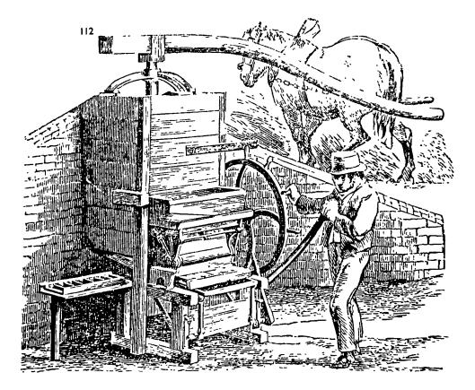
Figure 6.4. Hall's patent brick-moulding machine, British Patent No.10,845, 1845, Frederick Ransome, Assignee. [From <u>Catalogue Illustré des Machines et Instrumens Fabrique par</u>
