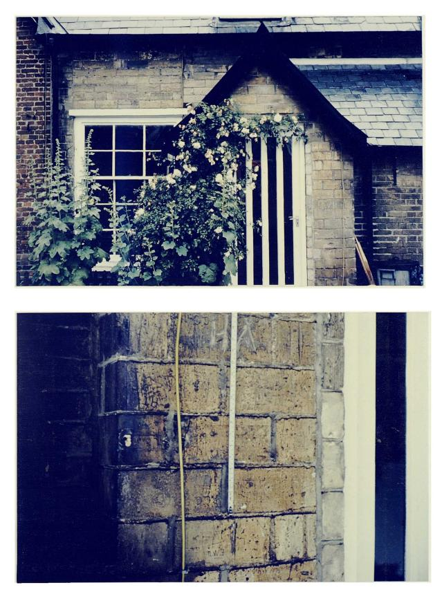
Figure 10.10.(top) and 10.11.(bottom) Porch constructed of hollow bricks in building at Banham, Norfolk (top). Close-up (bottom). [Photographs by author]
