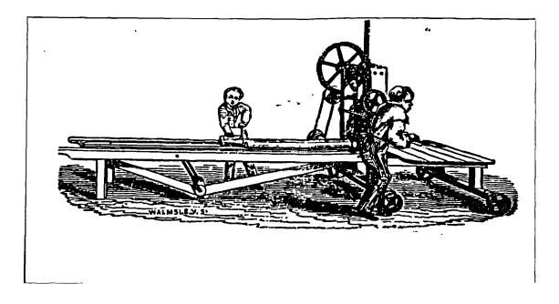
Figure 5.2. Unpatented tilemaking machine by John Hatcher of Benenden, Kent. [From trade catalogue, Cottam and Hallen, Winsley Street, Oxford Street, London, June 1847]
