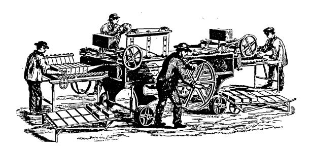
Figure 6.3. Clayton's "No. E" General Purpose Brick and Tile Machine. [From Henry Clayton, Son and Howlett trade catalogue, 1871]
