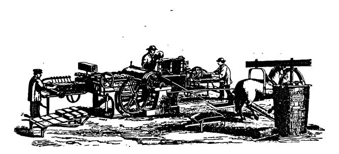
Figure 7.8. Henry Clayton's General Purpose "No. D" Brick and Tile Machine. [From Henry Clayton, Son & Howlett, <u>Atlas Works</u> (1871) p.32]
