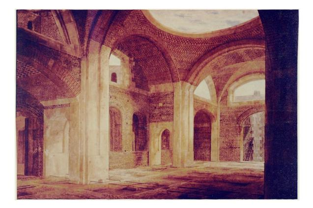
Figure 9.2. The Bank of England by John Soane; the Consol's Office before plastering, progress drawing by J. Gandy, 1799. [From John Summerson, <u>John Soane</u> (1983) p.72] Figure 9.3. The Bank of England by John Soane; vault of the Old Colonial or Five Per Cent Office, 1818, showing construction with earthenware cones, progress drawing by J. Gandy. [From John Summerson, John Soane (1983) p.69]
