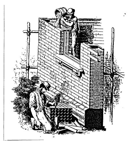
Figure 11.13. Construction of a concrete wall in stables and coach house at Hersham Lodge, Walton, Surrey using facing bricks manufactured by the Broomhall Tile Company. [From <u>The Builder</u> (1868) p.658]
