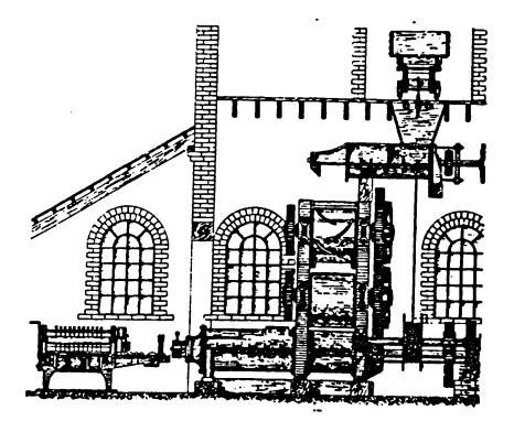
Figure 7.6. Extrusion brickmaking plant with feeder or trough mixer, two sets of crushing rolls, pug mill, die and cutting table. [From Alfred Searle, <u>Modern Brickmaking</u> (1931) p.139]
