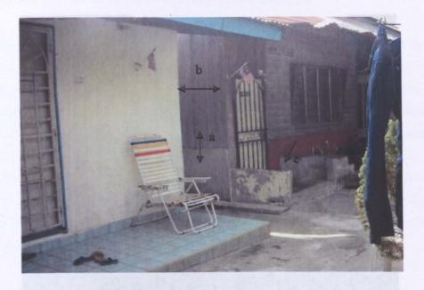
Figure 7.2. A typical house in Kampung Haji Abdullah Hukom. Note the mix of bricks and wood (see arrow a), the distance between the two houses (arrow b) and the protection against flooding in front one of the houses (arrow c).
