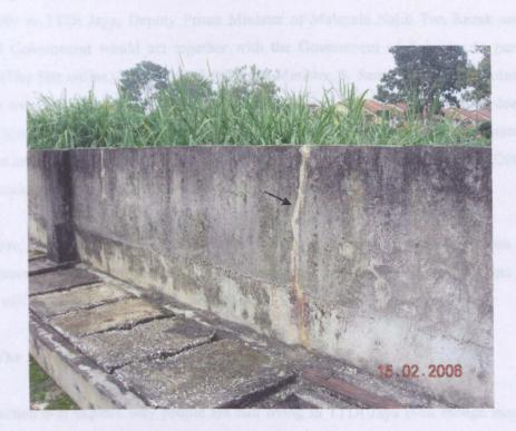
Figure 6.16. One of the cracks on the flood wall (see arrow).
