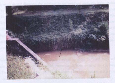
Figure 5.4a. A part of the Pantai River on which natural protection in the form of a barrier of branches was installed to control river bank erosion before 1998 (see arrow).
