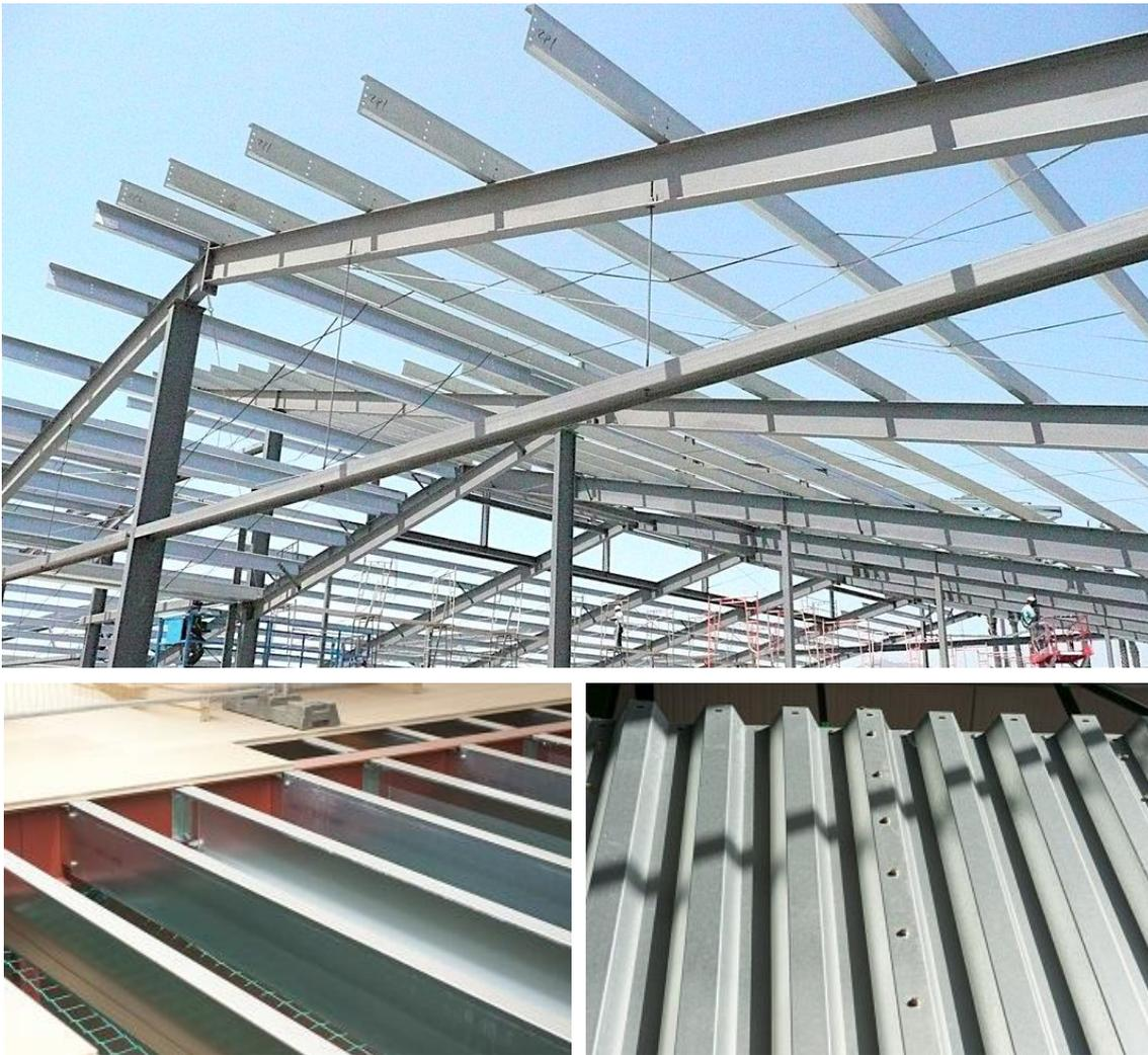
**Figure 1.1:** CFS used as secondary steelwork: a) roof purlins in a steel structure (<http://www.rki-bg.com> [accessed on August 2018]); b) beams in a mezzanine floor; c) wall cladding (<http://www.bw-industries.co.uk> [accessed on August 2018])
