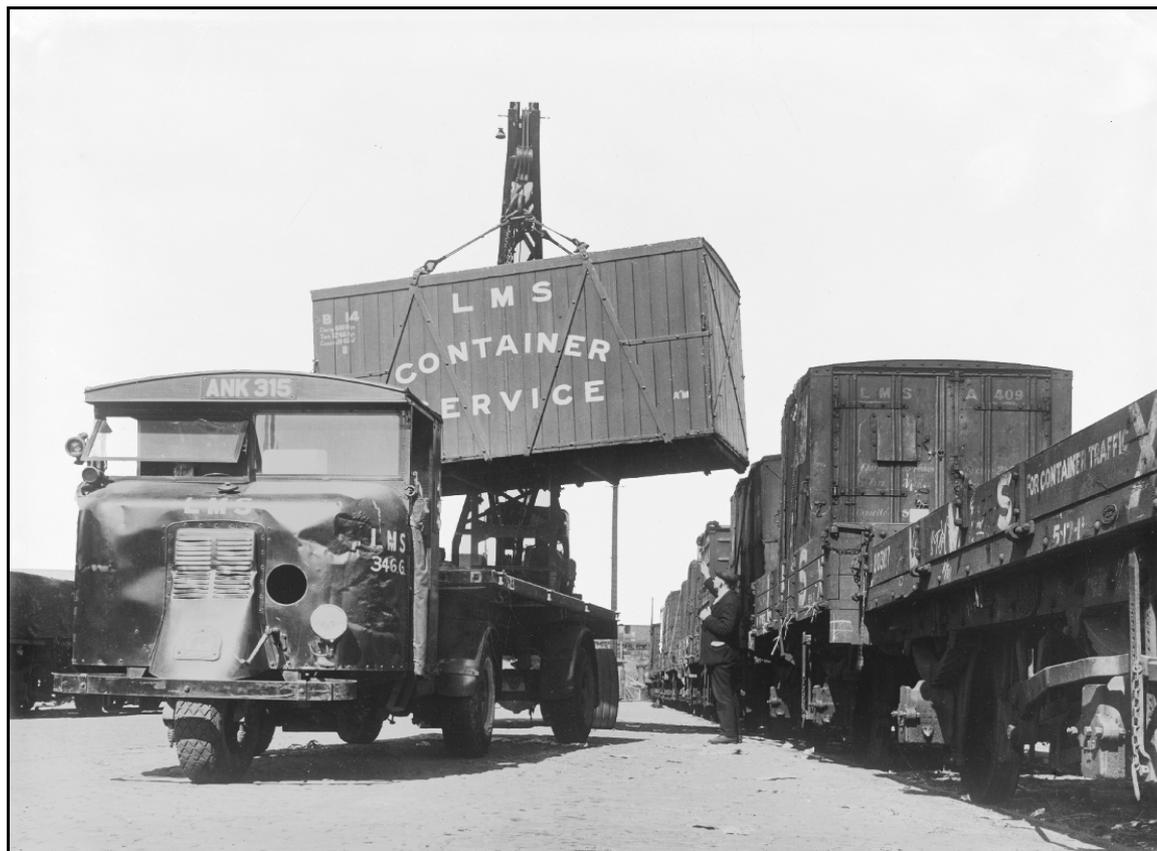
**An LMS container being transhipped in 1936. The photograph illustrates the degree of coordination between rail and road achieved by the railway companies following the container's introduction in 1926; the mechanical horse on the left is evidence of the LMS' ability to offer a complete door-to-door service to traders. One drawback to the scheme was the requirement for a mobile crane at every yard. Source: National Railway Museum 1997-7409\_LMS\_7933.**
