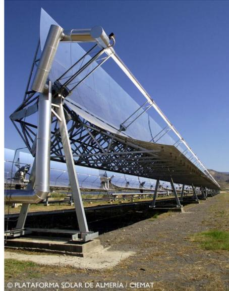
Figure F.1: ACUREX distributed solar collector field.
