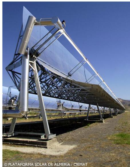
Figure 2.1: ACUREX distributed solar collector field.
