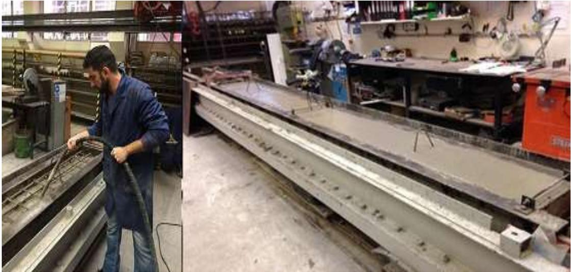
Figure 3-5: Using pocket vibrator during casting
