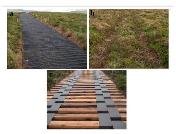
**Figure 5.1 a-c** Track types which have been included in this study. a) Plastic mesh, b) unsurfaced and c) articulated wooden.
