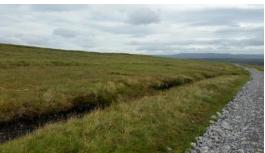
**Figure 4.9** Stone tracks with drainage channels running parallel to the track on the upslope side.
