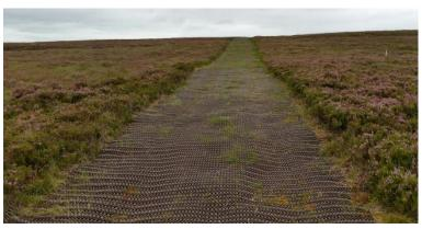
Figure 4.10 Plastic tracks installed perpendicular to the contours (i.e. straight up- and downslope) on working estates
