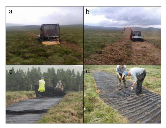
**Figure 3.8 a-d** a) Cutting of track route using a SOFTRAK with mower attachments, b) Removal of excess cut vegetation along track route using the SOFTRAK with forager attachment, c) Positioning of plastic mesh along route, and d) pinning of track route into place. Photos a) and b) courtesy of Alistair Lockett (North Pennines AONB Partnership).
