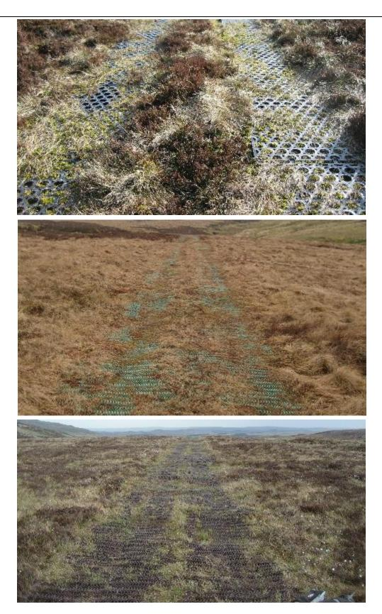
**Figure 4.2** Types of plastic track included in the regional survey. Top image of plastic boards used in three study reaches. Middle image 2 m wide plastic mesh and bottom image 2.5 m wide plastic mesh, both constructed from UPVC.
