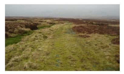
**Figure 8.2** Plastic mesh track, approximately 1 year after installation on a working estate where vegetation was not cut prior to installation.
