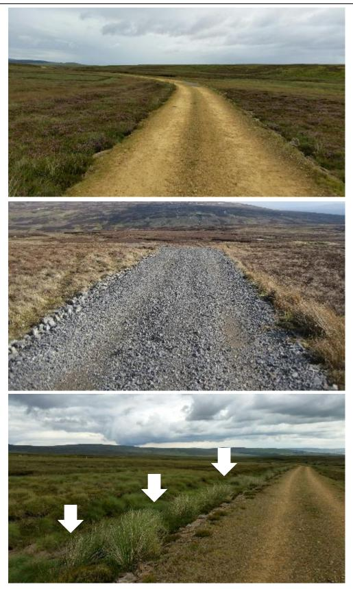
**Figure 4.3** Types of stone track included in the upland survey. Top image of a floating sandstone track. Middle image of a limestone floating track. Bottom image example of a borrow pit track, with excavation adjacent to the track (left of photo) indicated by the white arrows.
