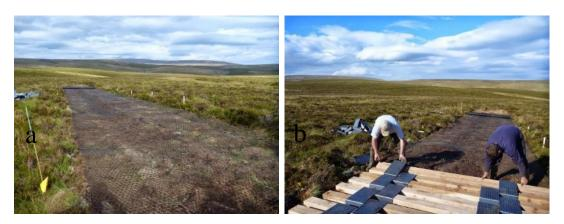
**Figure 3.9 a-b** Installation of wooden 4x4 track on Moor House NNR. a) Cut track route with thin plastic mesh and b) Oak beams laid along track route, connected with metal links. Photos courtesy of Andy Lloyd.
