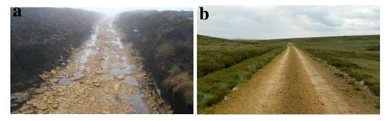
**Figure 2.3 a-b** a) Example of a 'cut and fill' road where the peat has been excavated and aggregate placed along the base of the trench to form the travelling surface. Photo Courtesy of North Pennines AONB. b) Example of floating road on blanket peat where the aggregate is placed on top of the peat surface.
