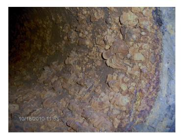
Figure 2.5: The internal surface of a  $\emptyset = 350$ mmm unlined DI trunk main, taken after the main had been drained down. Image supplied by Wessex Water.
